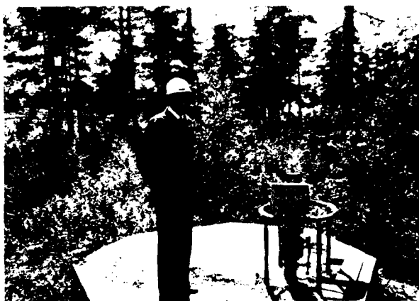
Photo 26. Vent installa- tion for underground cham- ber U-16, Skoeldvik Oil Refinery, Porvoo, Finland
