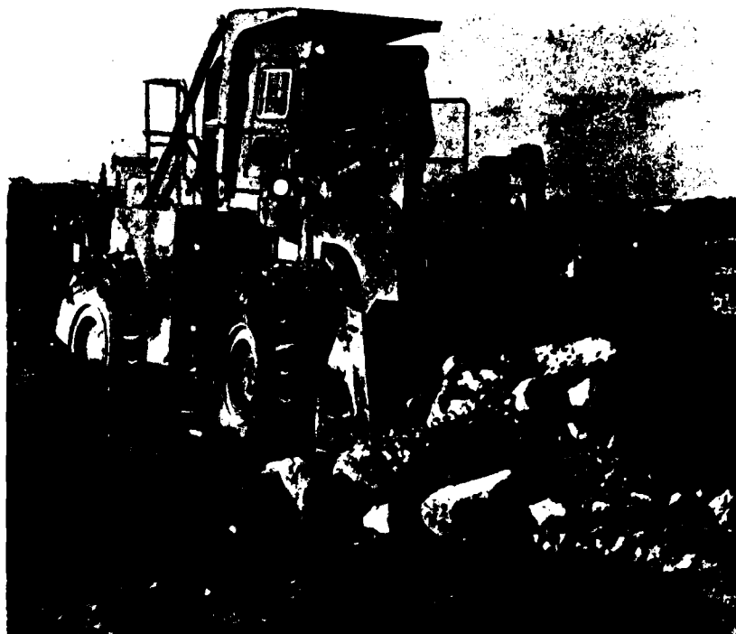
Photo 1. Selected size ejecta pushed into the crater and oversize to side of runway
