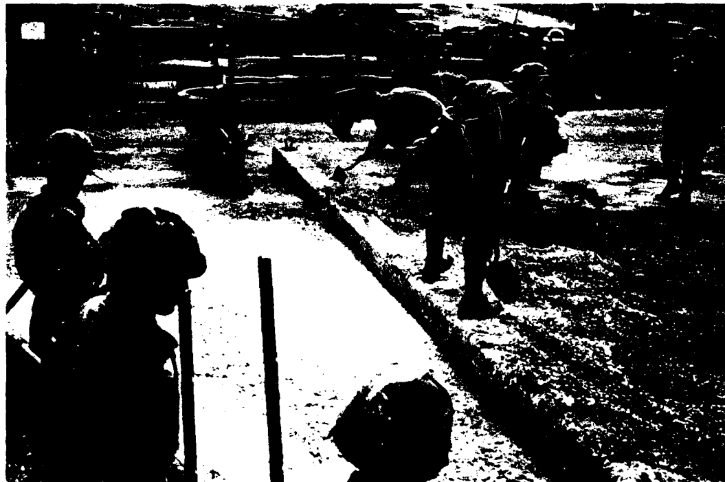
Photo 16. Sereel 1 and pulled forward to screed concrete flush with existing surface
