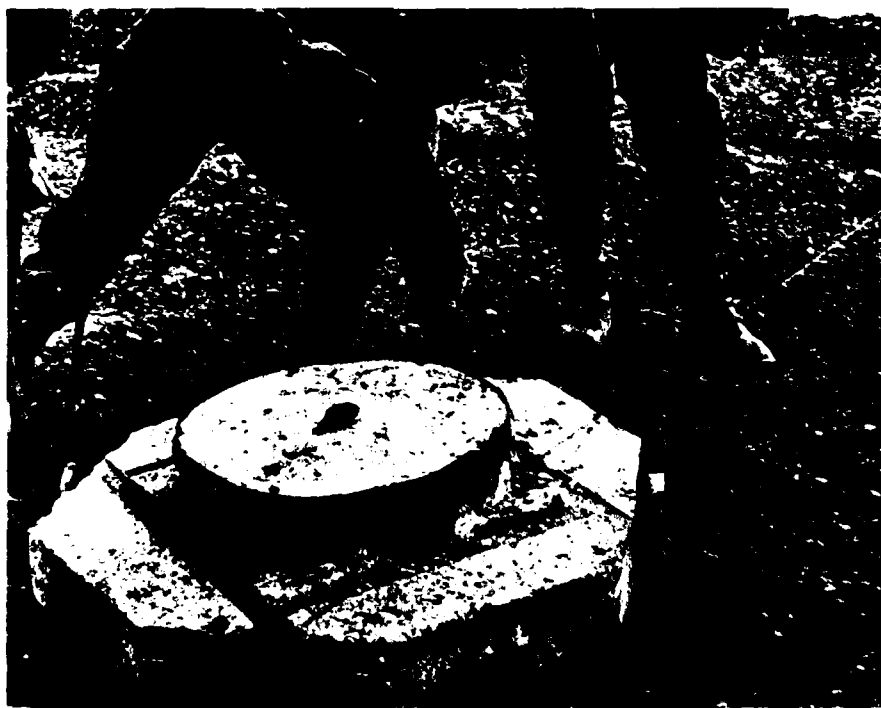
Photo 12. Screed pedestal placed in center of crater
