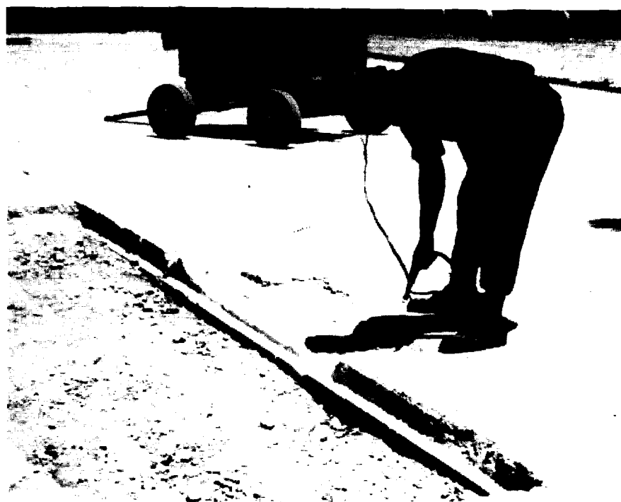
Figure 43. Cleaning the Pavement Edges With the Air Compressor
