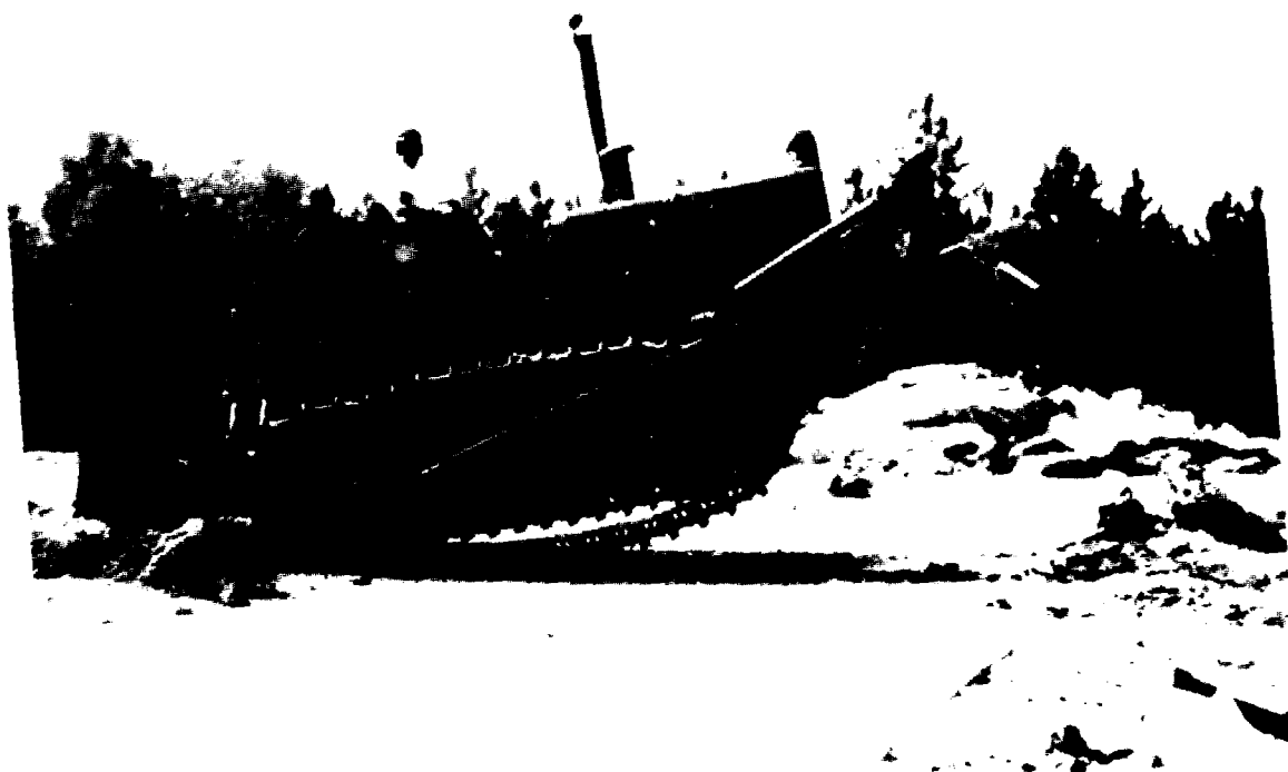
Figure 37. Dozer Too Small for Upheaval Removal
