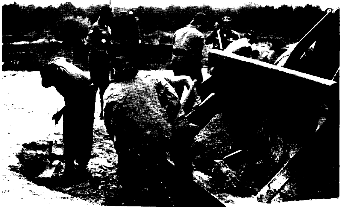
Figure 22. Cleaning the Debris Around the Crater Edges
