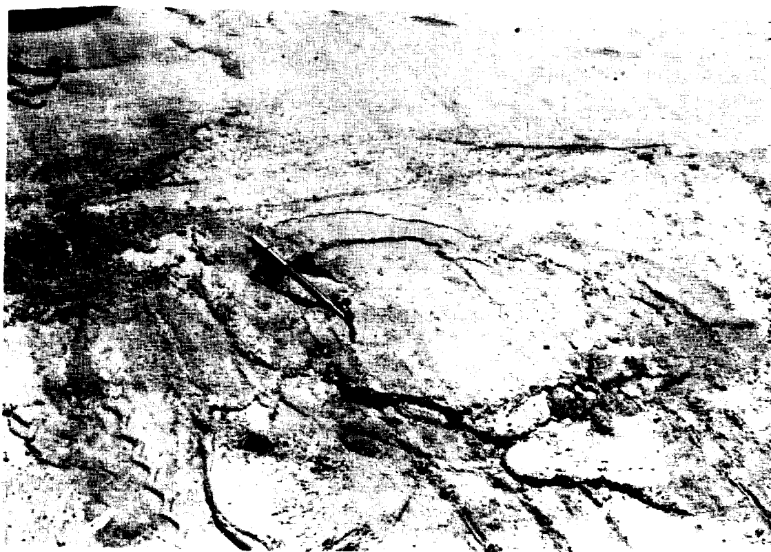
Figure 55. Quality Control Failure on Crater 4
