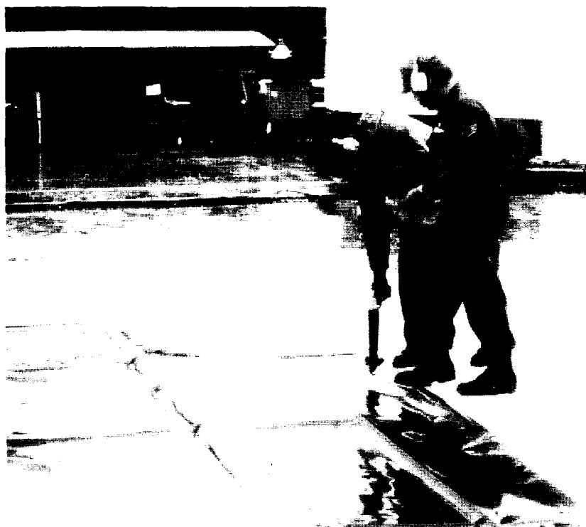
Figure 28. Anchoring the T-17 Membrane FOD Cover
