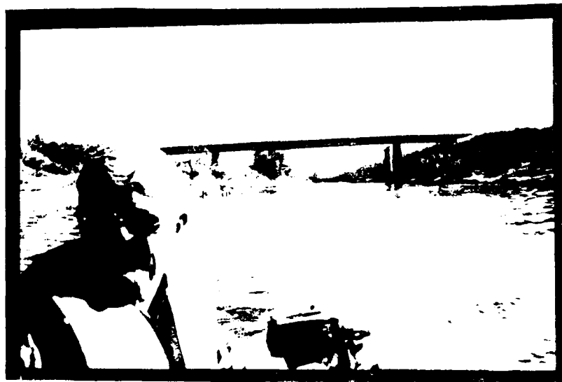
FIGURE B-15. SAMPLING SITE NO. 5. WESTMORELAND AVE BRIDGE
