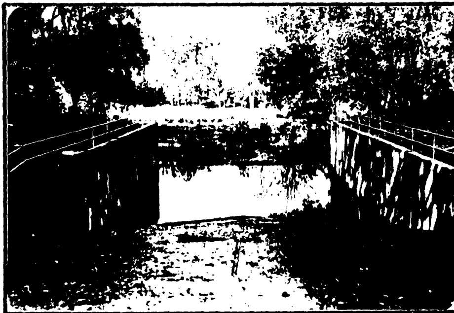
DOWNSTREAM CHANNEL - NO. 11 NOTE: TILTED WALL
