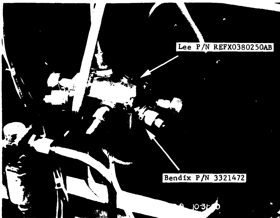
FIGURE 26. LHS solenoid valve and restrictor
