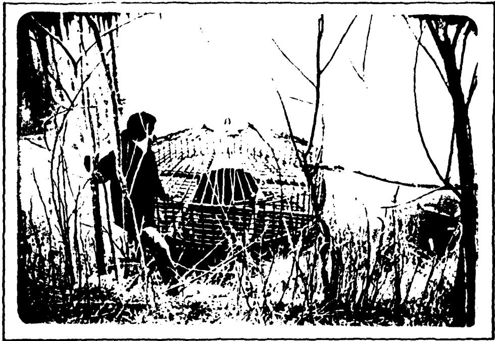
3. NORMAL OVLRFLOW SPILLWAY ENTRANCE WITH STEEL ROD TRASHRACK .(12/15/80)
