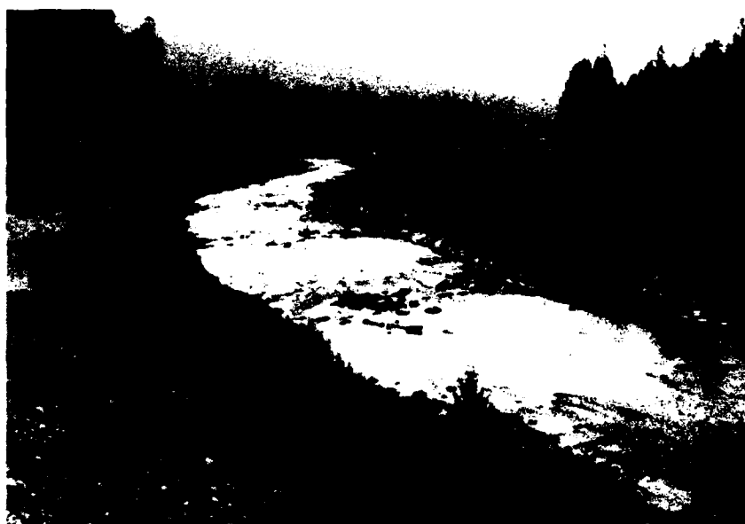
b. The groins were still recognizable on the date of the WES inspection visit (8 Aug 79); however, the rock was widely scattered
