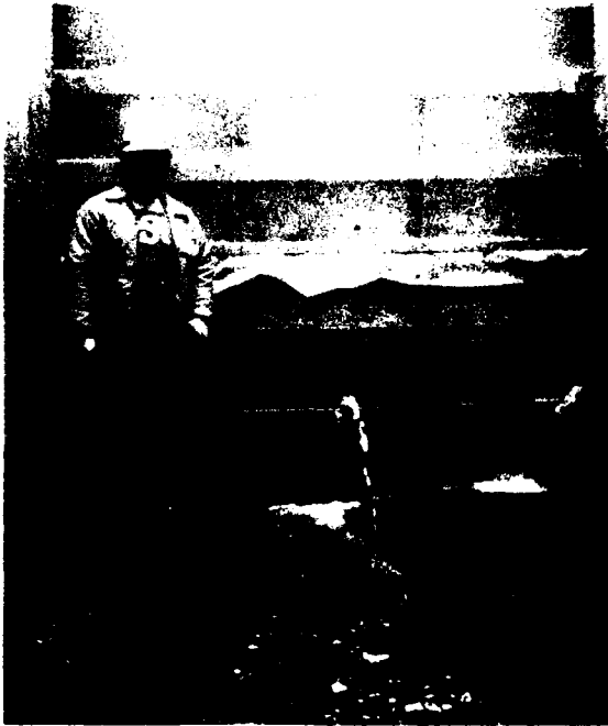
Photo No. 3. Leakage past stoplogs with stream level approximately 2 ft. above intake invert.
