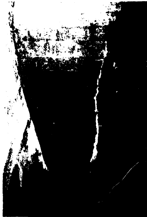
Photo No. 4. Crack in top of transition section of intake structure.
