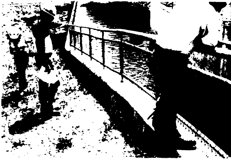
Photo No. 5. Displacement of stilling basin posts and handrails - left side.
