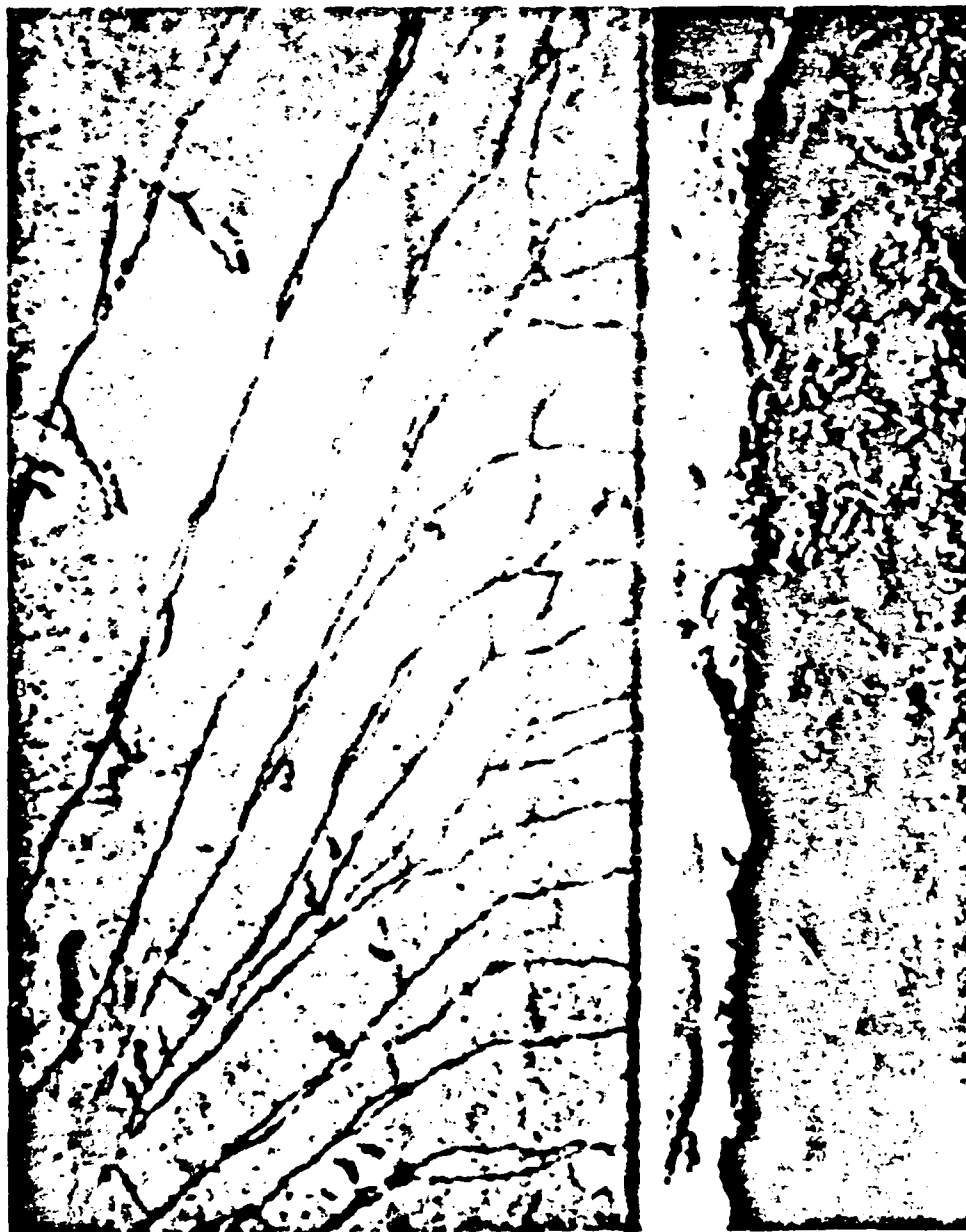
FIG. 45: Diagonal Cracking
