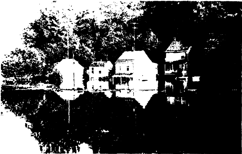
FIGURE 6 - Bushkill Drive at Easton, Pennsylvania, as it appeared during the flood of 18-19 August 1955. Note floating debris in center of photograph.
