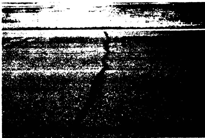
Figure 1. Sealed reflective cracks (runway 16-34, Great Falls)
