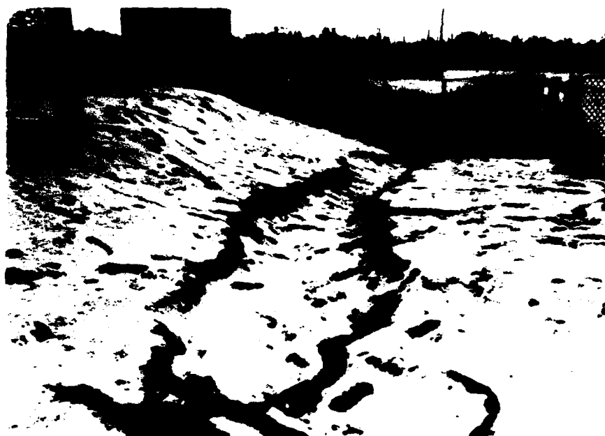
Photo 5 - View of erosion on left bank of channel between the old and new bridges at the concrete weir spillway. (Photo taken January 14, 1981).
