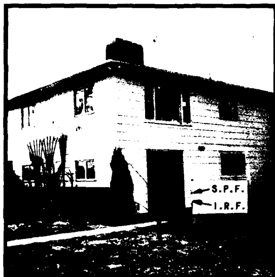
Figure 39. KOEPEL ROAD - TONAWANDA CREEK Arrows indicate the height of the Standard Project and Intermediate Regional Floods at a Koepsel Rd. residence located near mile 36.5 along Tonawanda Creek.
