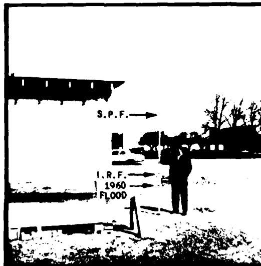
Figure 38. PARK AND MARINA - TONAWANDA CREEK. The flood heights for the Standard Project, Intermediate Regional and the 1960 flood are shown at the Niagara County West Canal Park and Marina near mile 5.2 along Tonawanda Creek.
