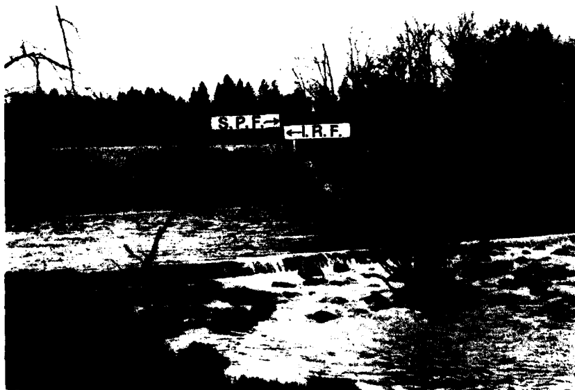
FIGURE 31 — Heights of flooding at Hinckley Lake dam, river mile 36.49 are shown by the arrows for the Standard Project and Intermediate Regional Floods.
