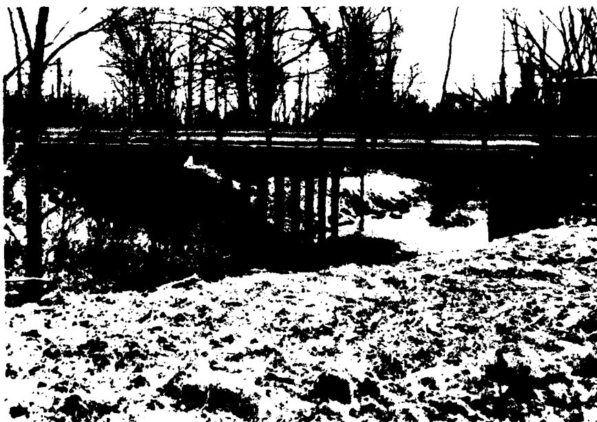
FIGURE 25 — View of downstream face of Route 303 bridge at river mile 35.32.
