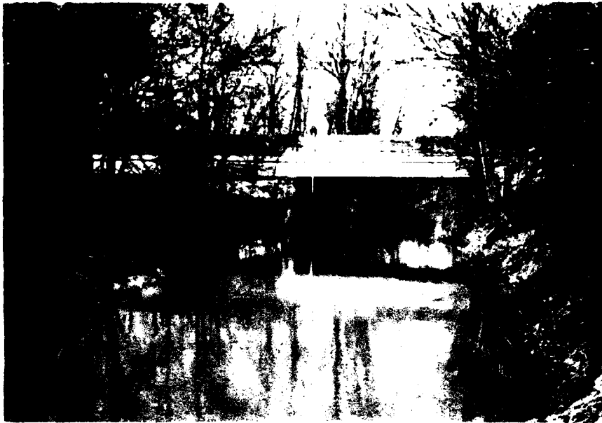
FIGURE 20 — Looking downstream at upstream face of Bennett Road bridge at river mile 28.43.
