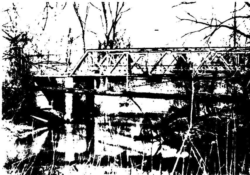
FIGURE 23 — Boston Road bridge at river mile 31.15. Looking downstream at upstream face.
