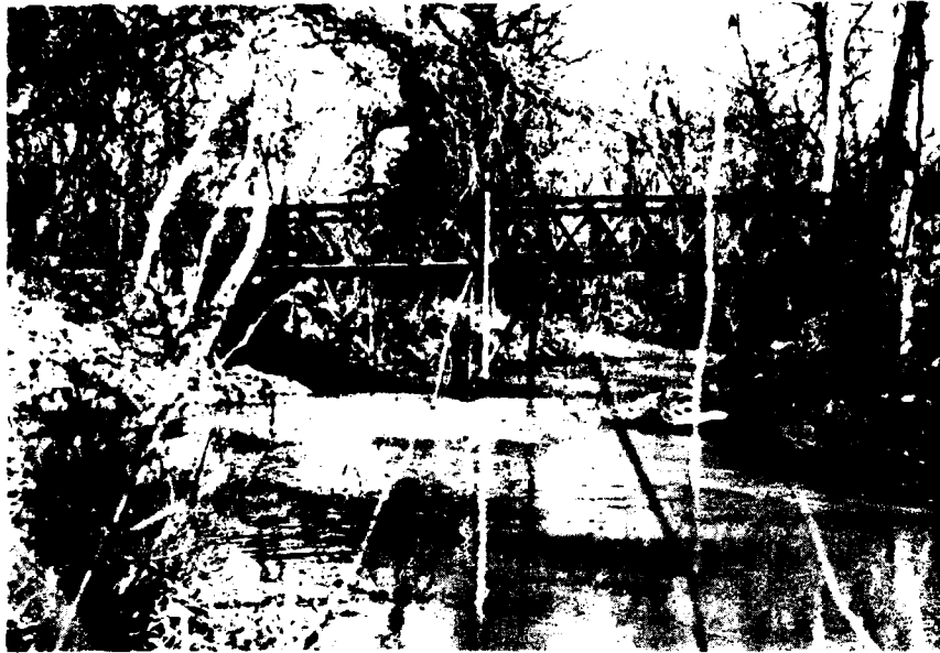
FIGURE 22 — View of private road bridge looking upstream at river mile 20.78.
