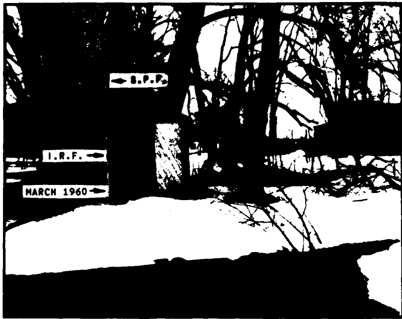
Figure 12 - Arrows indicate the heights of the Standard Project, Intermediate Regional, and March 1960 floods, stream mile 0.5.
