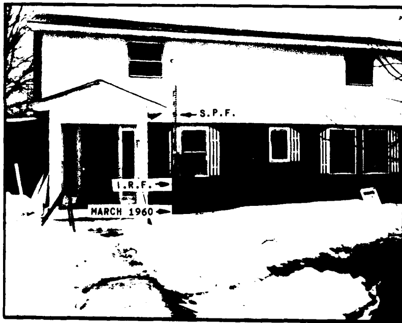
Figure 13 - Arrows indicate the heights of the Standard Project, Intermediate Regional, and March 1960 floods at residence on Hitchcock Road, stream mile 1.8.
