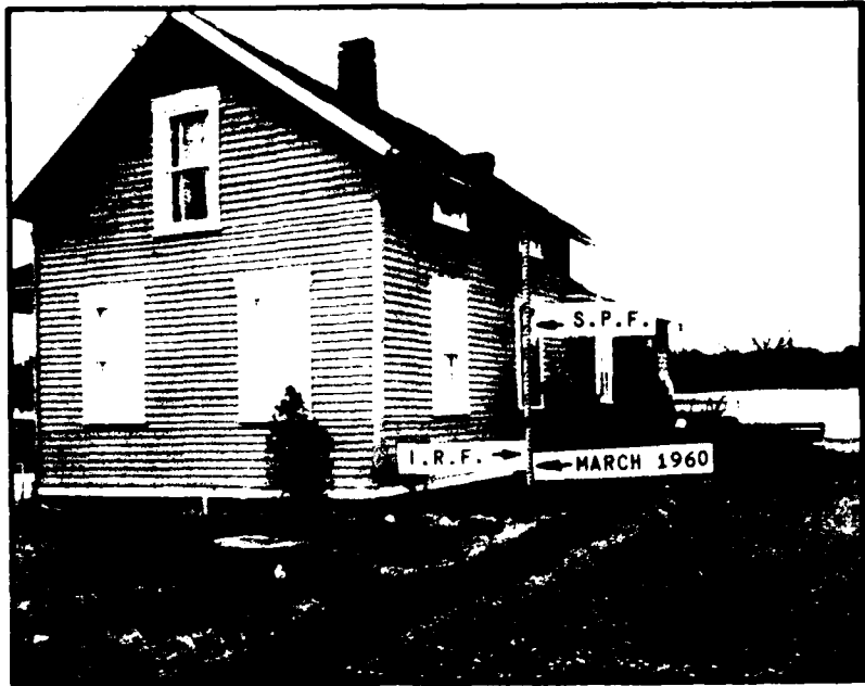
Figure 16 - Arrows indicate the heights of the Standard Project, Intermediate Regional, and March 1960 floods at residence on N.Y.S. Route 298, stream mile 4.7.
