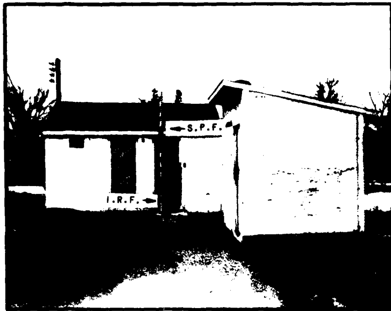
Figure 14 - Arrows indicate the heights of the Standard Project and Intermediate Regional floods at pump house just downstream of N.Y.S. Route 31, stream mile 3.4.
