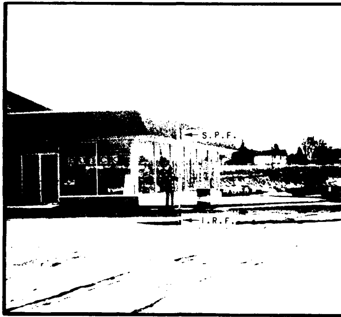
Figure 29 Arrows indicate the heights of the Intermediate Regional and the Standard Project floods at a car dealer on the downstream side of East Main Street bridge, stream mile 1.59. Photograph taken in January 1972.
