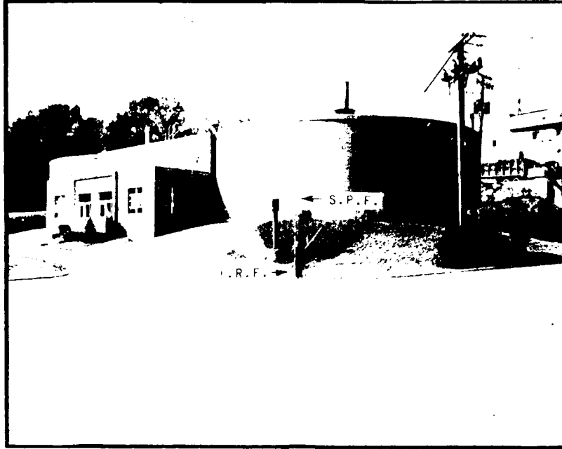
Figure 25 Arrows indicate the heights of the Intermediate Regional and the Standard Project floods at Sewage treatment plant, stream mile 54.0.
