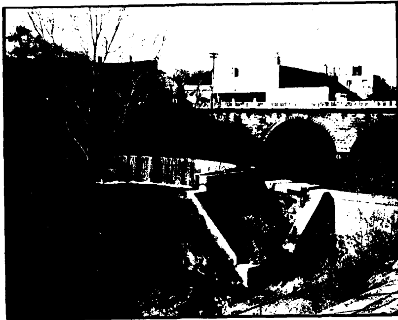
Figure 18 Looking upstream at Dam located at stream mile 54.96. West Main Street is in the background. Photograph taken in November 1971.
