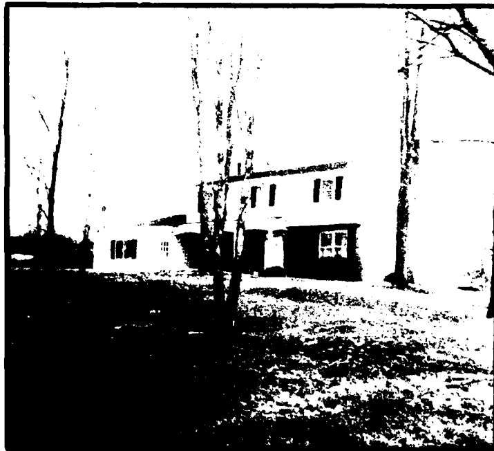
Figure 24 House, bordering Breakneck Creek at stream mile 3.05, built up to be well out of the range of the Intermediate Regional Flood or the Standard Project Flood. Photographs taken in February 1972.
