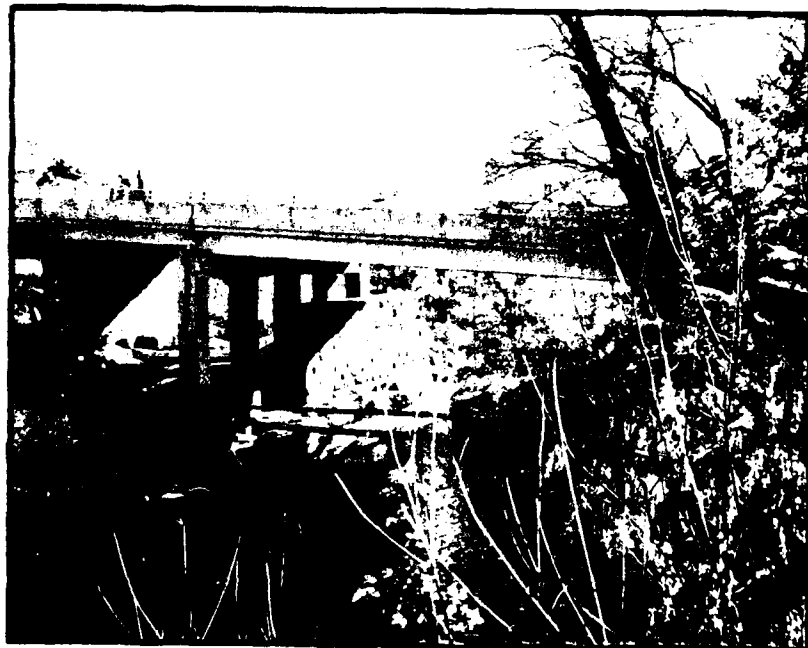
Figure 9 upstream face of Crain Avenue bridge, stream mile 55.35. Note pipelines which are obstructions to high flows.
