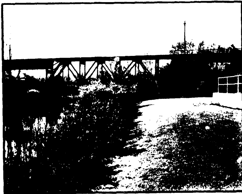
Figure 3 Upstream face of Norfolk and Western Rail- way bridge, stream mile 53.95.
