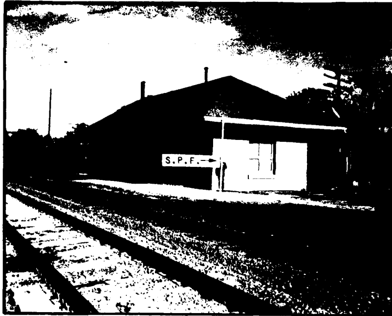
Figure 23 Low damage development which is compatible with wise flood plain useage. Arrow indicates the height of the Standard Project Flood Stream mile 54.58. Photograph taken in November 1971.
