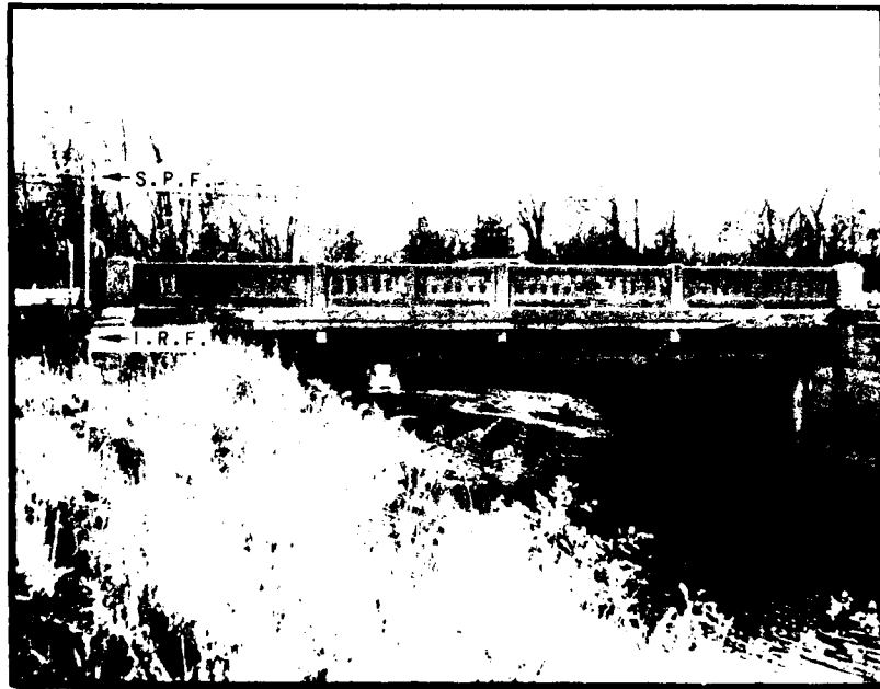
Figure 30 Arrows indicate the heights of the Intermediate Regional and the Standard Project floods at the East Main Street bridge, stream mile 1.6. Photograph taken in November 1971.
