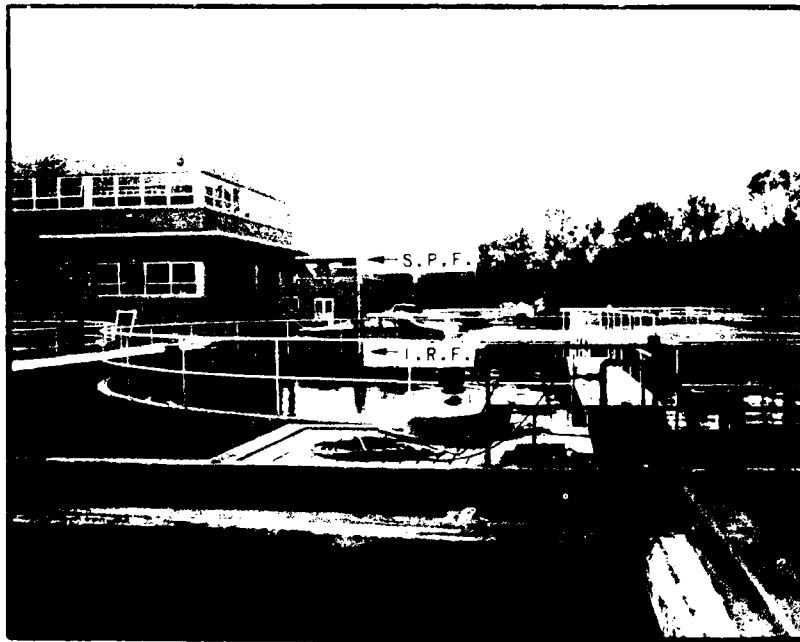
Figure 26 Arrows indicate the heights of the Intermediate Regional and the Standard Project floods at Sewage treatment plant, stream mile 54.0.
