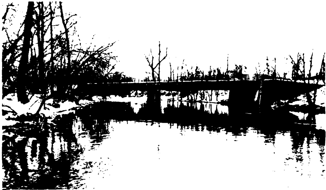
Figure 5 – View of upstream side of Bowerman Road bridge, creek mile point 2.60. Photo taken February 1973.
