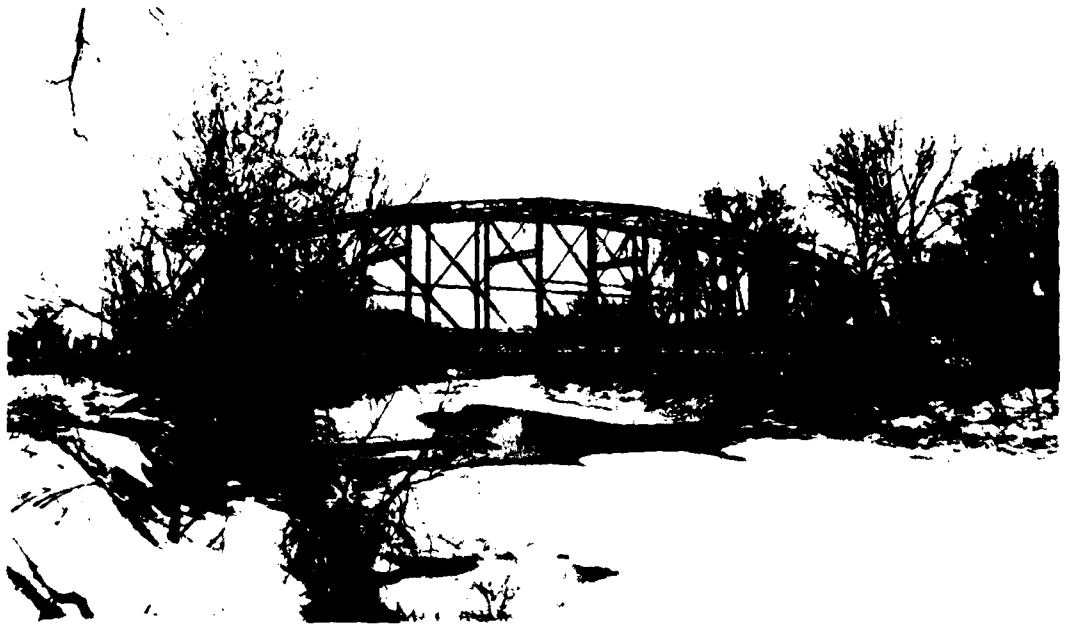
Figure 2 – View of upstream side of Rush Road bridge, river mile point 23.90. Photo taken February 1973.
