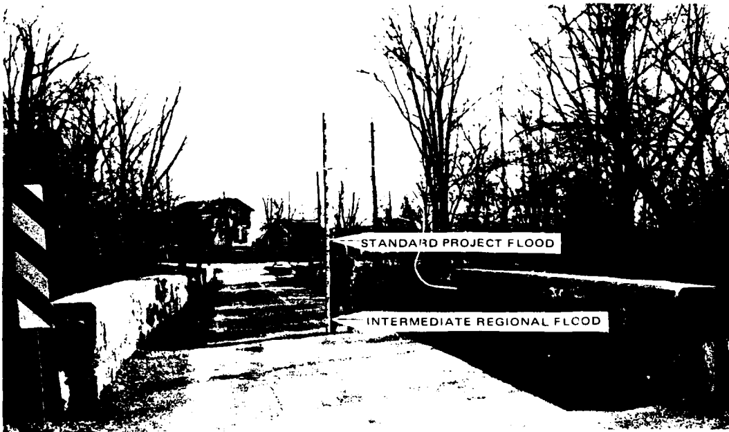
Figure 15 - Future flood heights at State Street bridge near Mumford. Photo taken January 1973.
