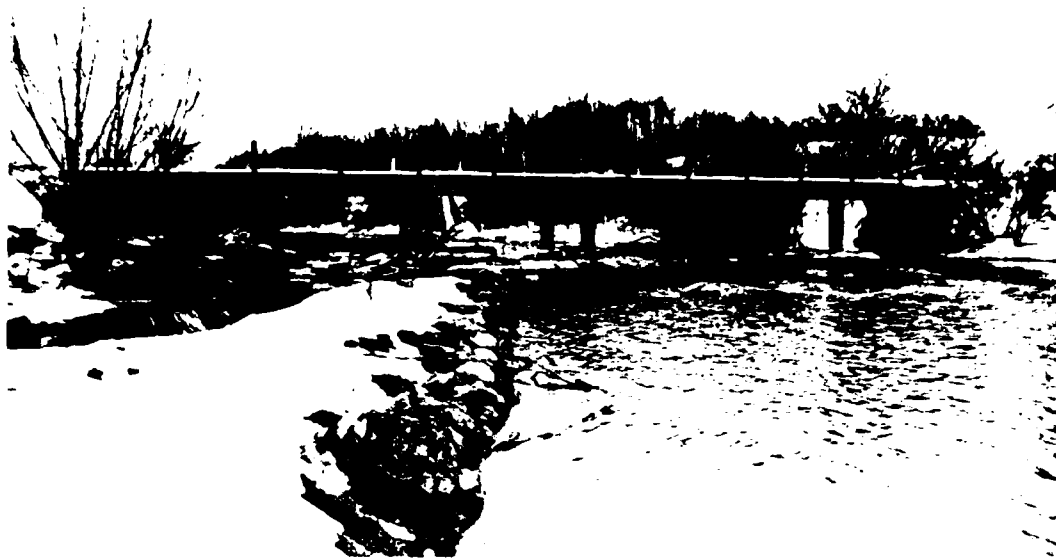
Figure 7 – View of upstream side of private access bridge, creek mile point 4.70. Photo taken February 1973.
