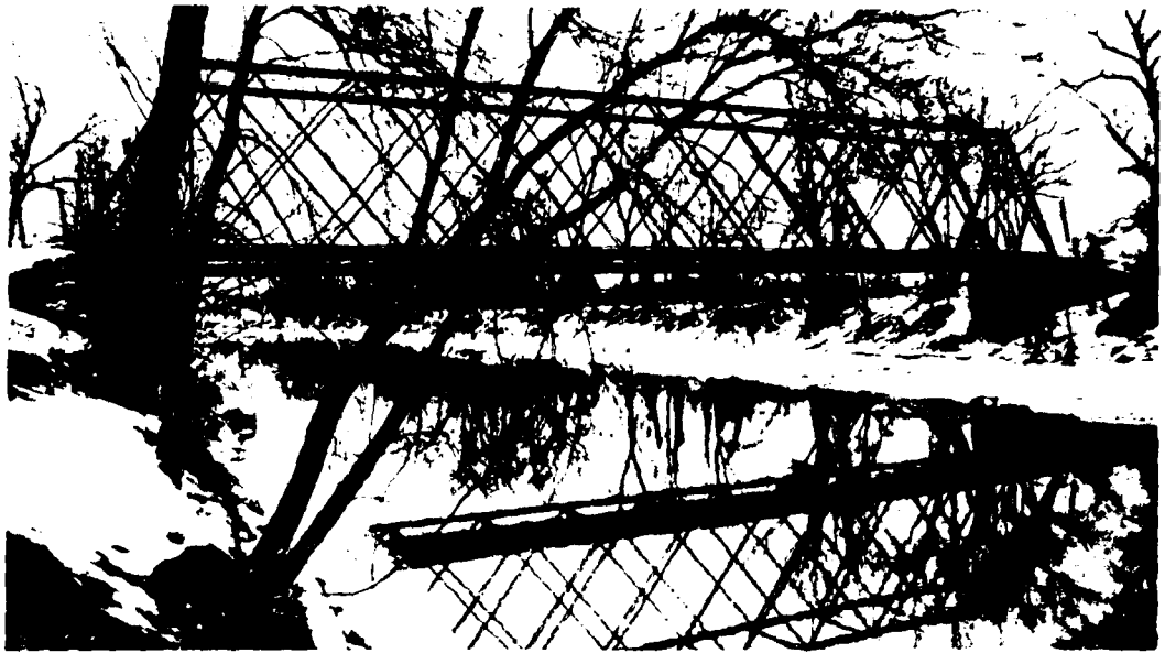
Figure 1 – View of upstream side of Scottsville - Henrietta Road bridge, river mile point 21.70. Photo taken February 1973.
