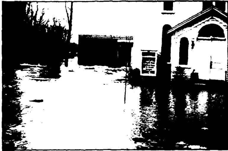
Photo No. 13. Elma Methodist Church and Sunday School addition on Bowen Road, during the March 1962 flood.
