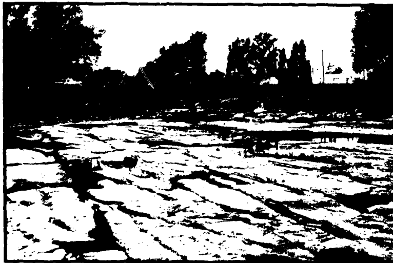
Photo No. 20. Looking downstream at Transit Road bridge showing the rock channel bottom.
