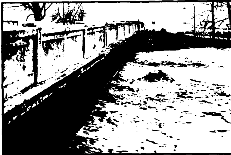
Photo No. 7. Looking south from the north abutment at the downstream side of the Transit Road bridge during the March 1955 flood.
