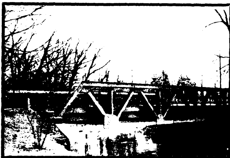
Figure 4 - View looking upstream at Pavement Road Bridge.
