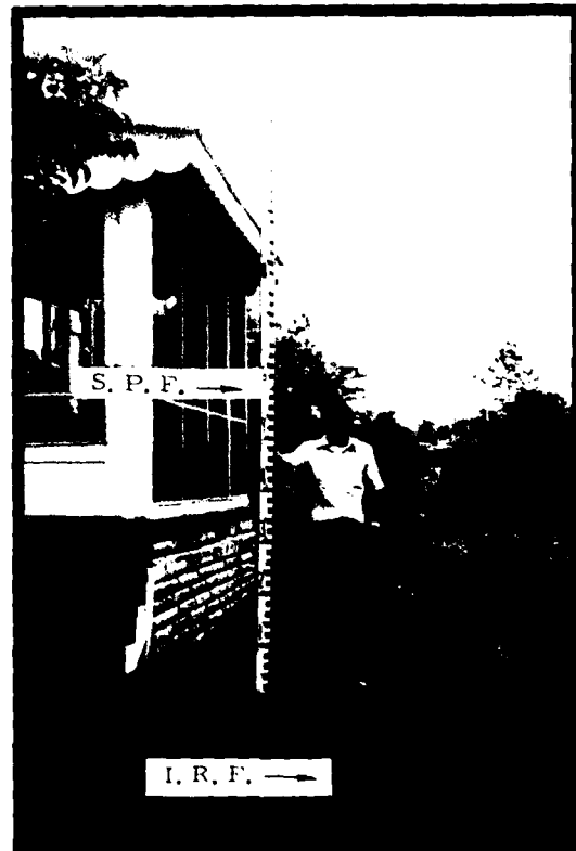
Figure 22 - Photo showing Standard Project Flood height at an existing building on Townline Road, Lancaster, New York. The building would be half submerged under such a flood. Intermediate Regional Flood elevation also is shown.
