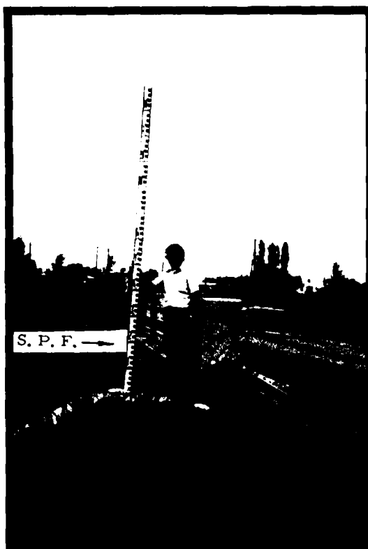
Figure 20 - This picture shows that the roadway of the Crittenden Road bridge in the Village of Alden would be almost submerged from the Standard Project Flood.
