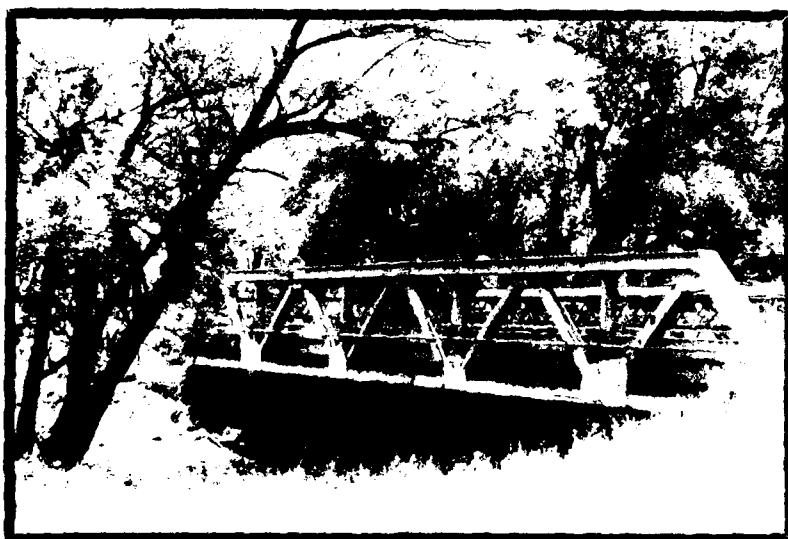
Figure 5 - View looking downstream at Pavement Road Bridge. The bridge deck is very low with respect to the stream bed so that even moderate flooding would overflow the road.
