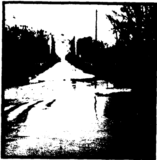
Figure 17 - Flooding conditions on 29 January 1970 at Grafton Road bridge, stream mile 28.02.
