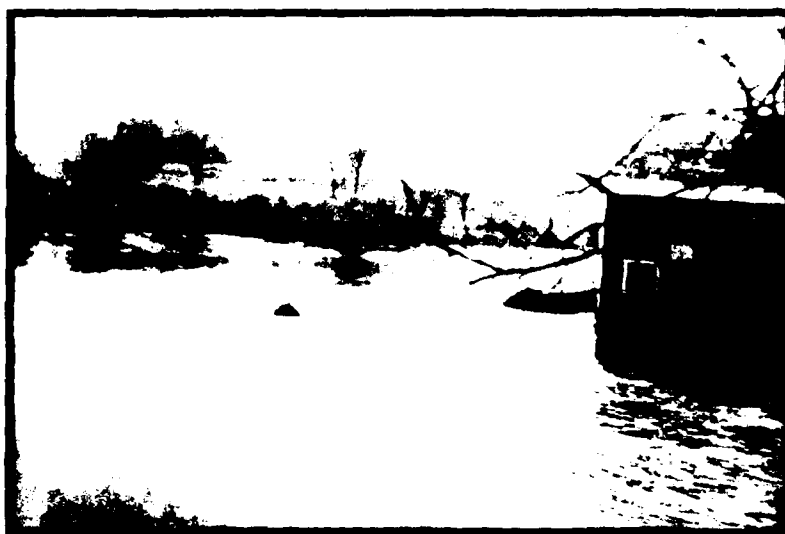
Figure 19 - 1938 high water conditions at Nichols Road, stream mile 45.87.
