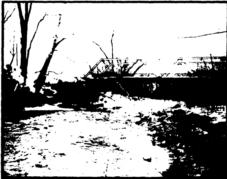
Figure 11 - Looking downstream at Bagdad Road bridge, stream mile 43.10.
