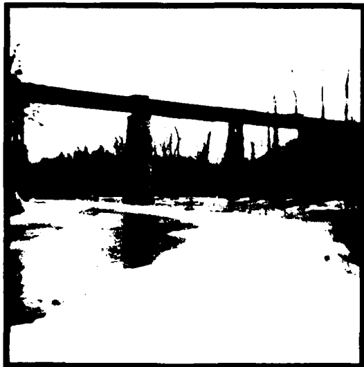
Figure 9 - Looking downstream at Baltimore & Ohio Railroad bridge, stream mile 32.75.
