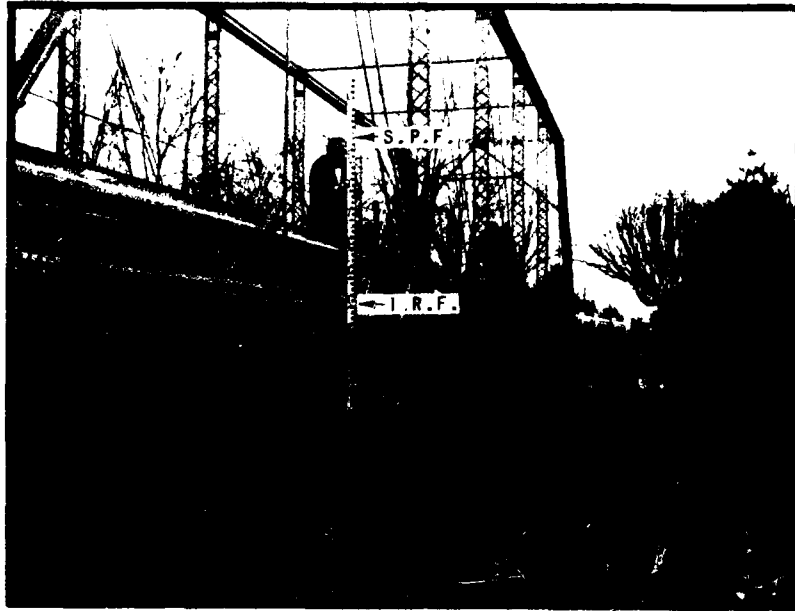
Figure 21 - Arrows indicate the heights of the Standard Project and Intermediate Regional Floods at Grafton Road bridge, stream mile 28.02. Photo taken March 1970.
