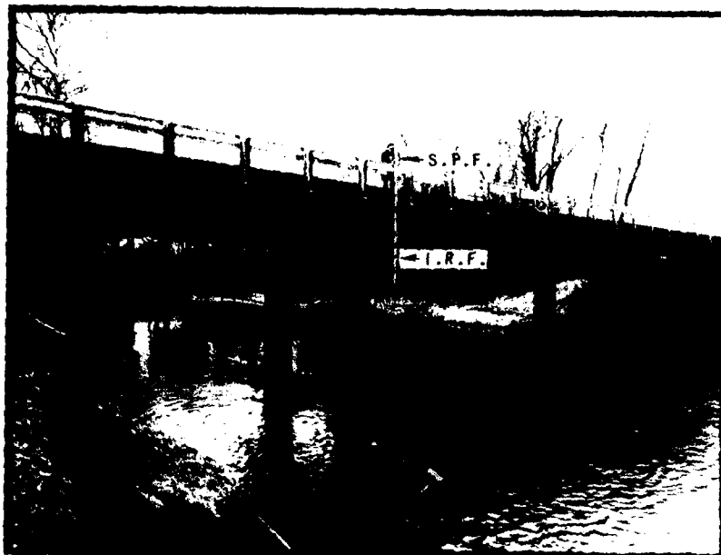
Figure 23 - Arrows indicate the heights of the Standard Project and Intermediate Regional Floods at Ohio State Route 252 bridge, stream mile 31.53. Photo taken March 1970.
