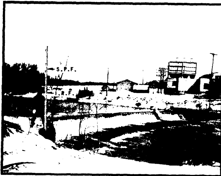
Figure 27 - Arrows indicate the heights of the Standard Project and Intermediate Regional Floods at the dam adjacent to the Medina City Waterworks, stream mile 42.0.
