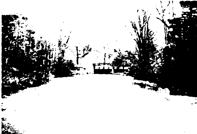
FIGURE 1 - Railroad bridge abutments can cause stream to back up (Nov. 9, 1972)
