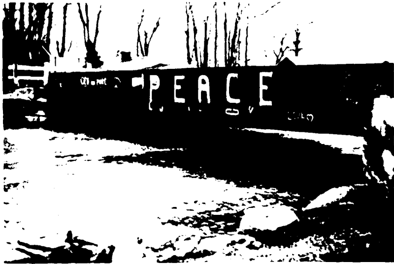
FIGURE 13 - Lake Road Bridge at mouth of Oneida Creek (Nov. 9, 1972)
