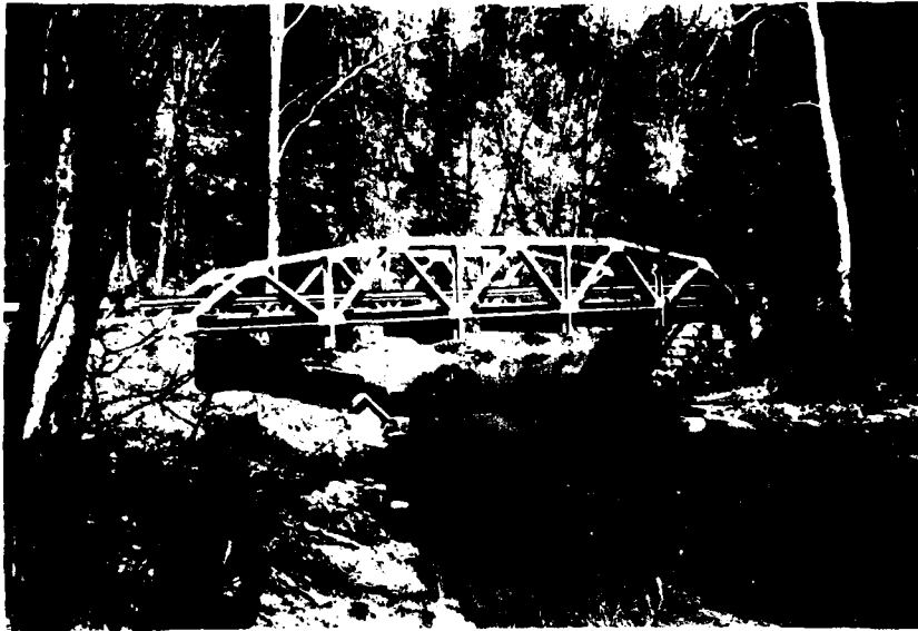
Figure 9 - Upstream view of Wisner Road Bridge at stream mile 12.01.
