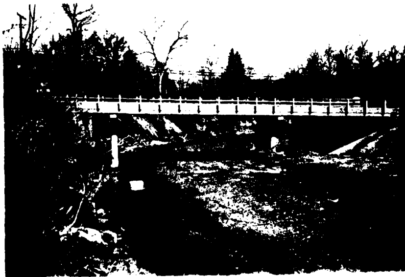
Figure 6 - Upstream view of the Chillicothe Road Bridge at stream mile 3.72.
