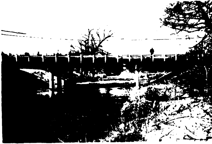
Figure 5 - Upstream view of the Route 306 Bridge at stream mile 2.97.
