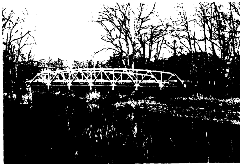
Figure 4 - Upstream view of the Markell Road Bridge at stream mile 2.52.
