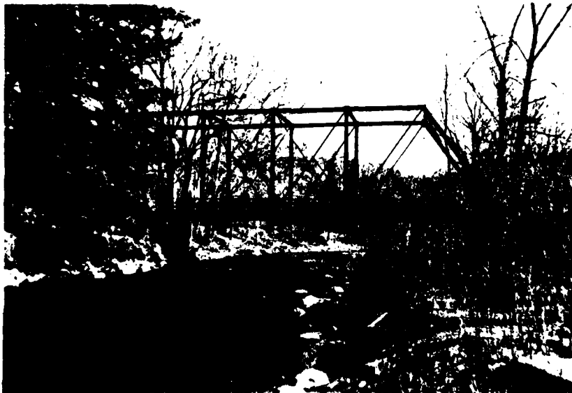
Figure 8 - Upstream view of Mitchells Mill Road Bridge at stream mile 10.81.
