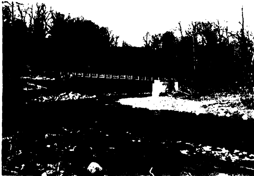
Figure 7 - Upstream view of Booth Road Bridge at stream mile 6.93.
