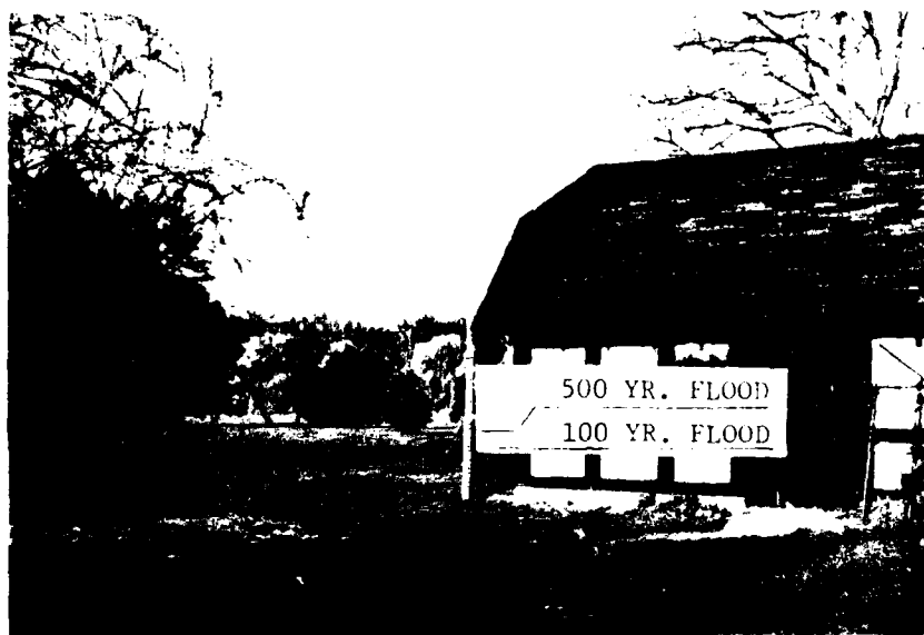
Figure 15 - The 100 and 500 year flood heights on the Pump house at the Kirtland Country Club at stream mile 2.12.
