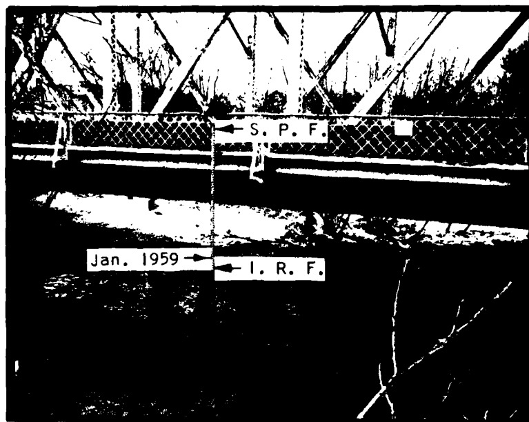
Figure 29 - Arrows indicate the heights of the Standard Project, Intermediate Regional, and the January 1959 floods at the upstream face of the Akron-Peninsula Road bridge, stream mile 40.25.
