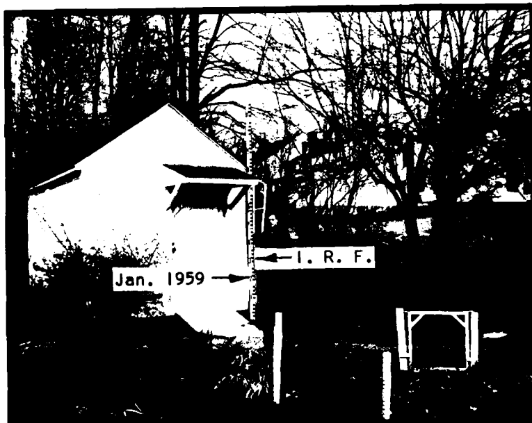
Figure 34 - Arrows indicate the heights of the Intermediate Regional and the January 1959 floods along South Park Drive in the Village of Silver Lake, stream mile 47.95.
