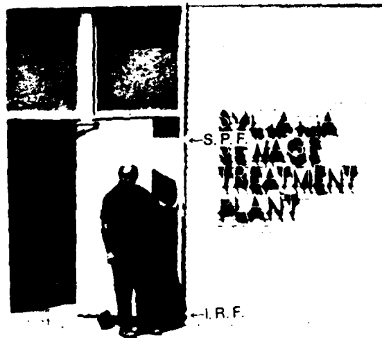
Sylvania Sewage Treatment Plant at river mile 19.86.
