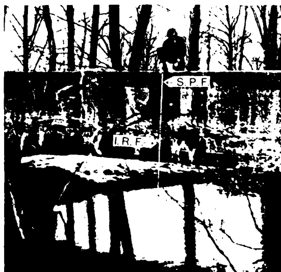
Brint Road Bridge at river mile 23.03.
