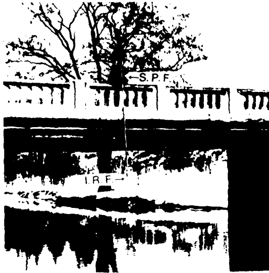
Sturbridge Road Bridge at river mile 17.65.
