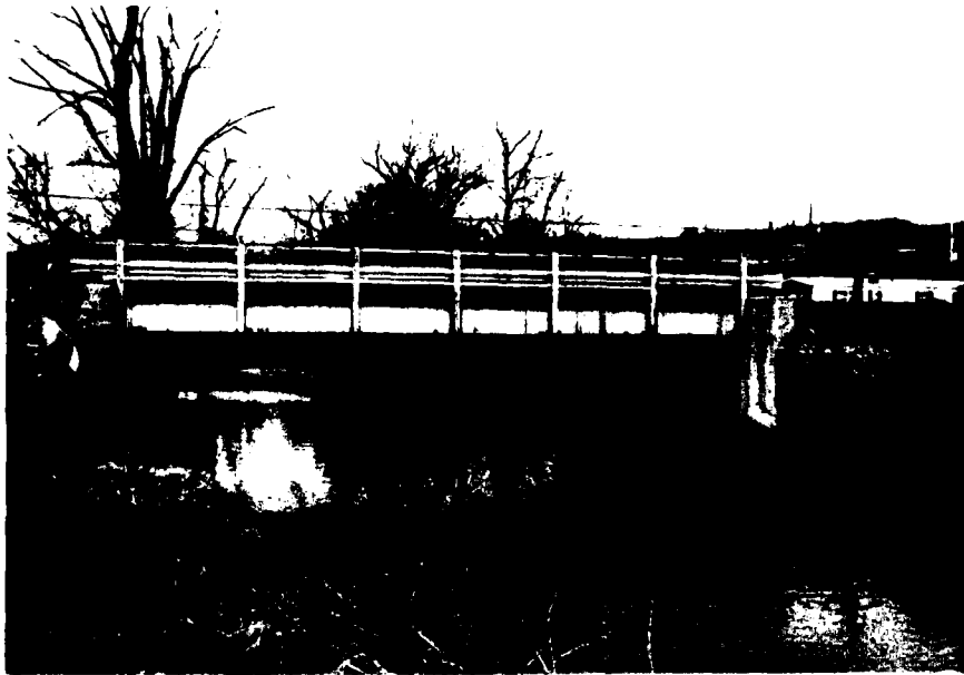
Figure 10 - Upstream face of the Cat Path Road bridge at Stream Mile 9.45.
