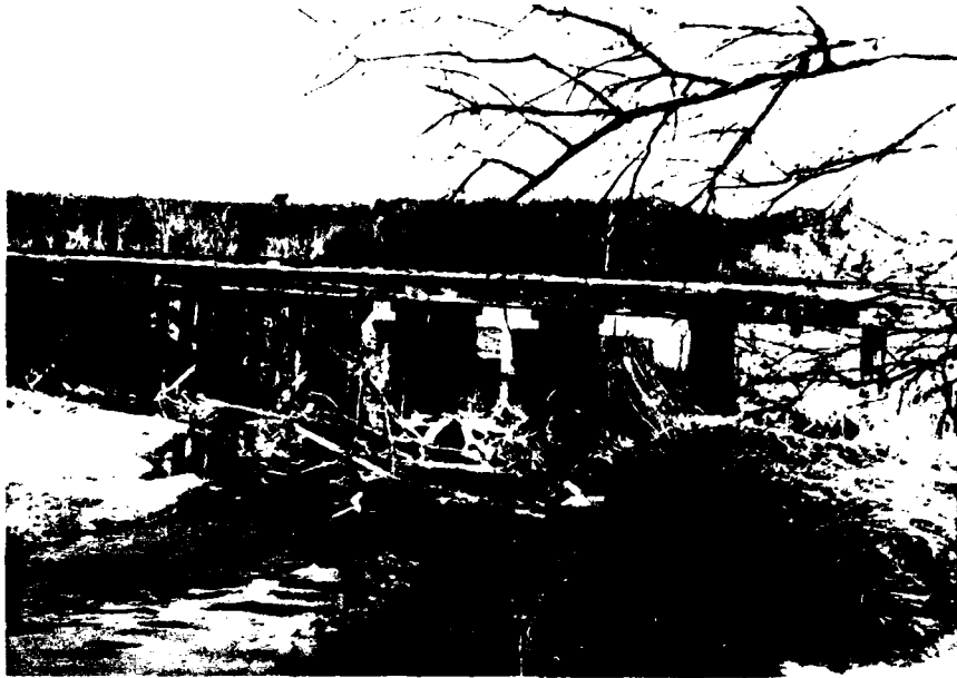
Figure 2 - Upstream face of the Lehigh Valley Railroad Bridge at Stream Mile 9.31. Note debris at face of bridge. Route 38 bridge in background.
