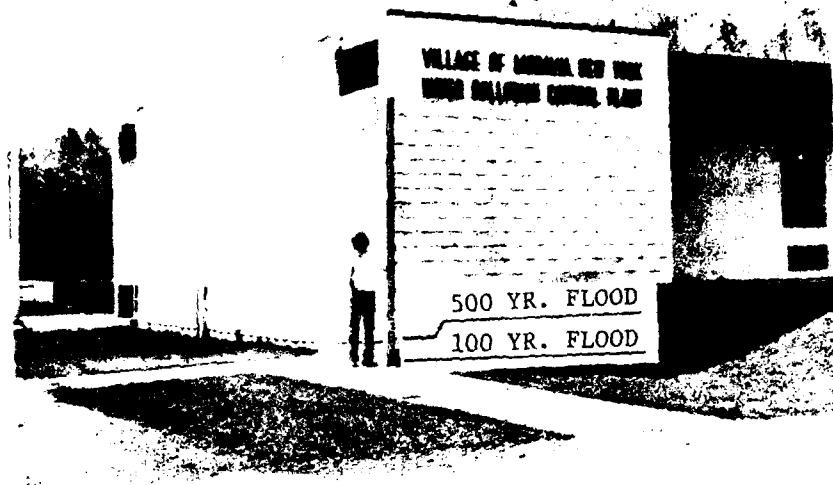
Figure 15 - Future flood heights at village of Moravia Water Pollution Control Plant, Stream Mile 4.5.
