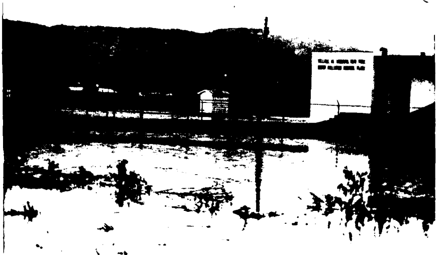
Figure 14 - Flooding conditions at village of Moravia Water Pollution Control Plant, on Long Hill Road during September 1975 high water. Stream Mile 4.5.
