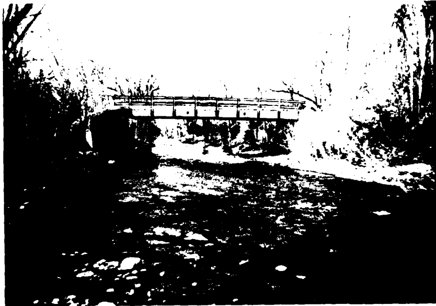
Figure 8 - Upstream face of the Erron Hill Road bridge, Stream Mile 8.4.
