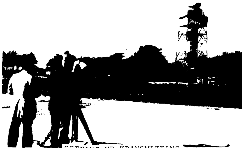
SETTING-UP TRANSMITTING ANTENNA ON PAD #1
