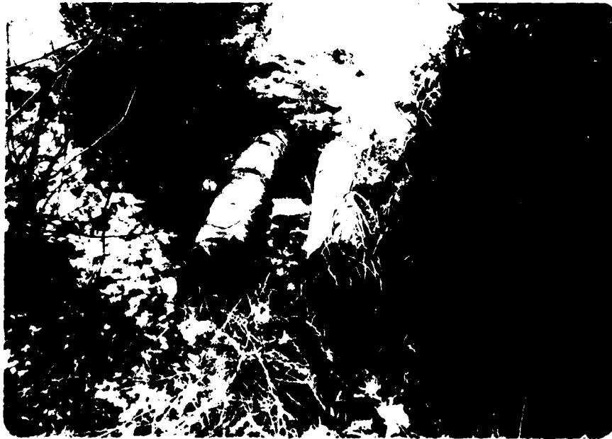
Photo 6 - View of discharge end of 12-inch C.M.P. Flow is from the pipe on the right. Upstream end of pipe on the left could not be found. (Photo taken January 14, 1981).
