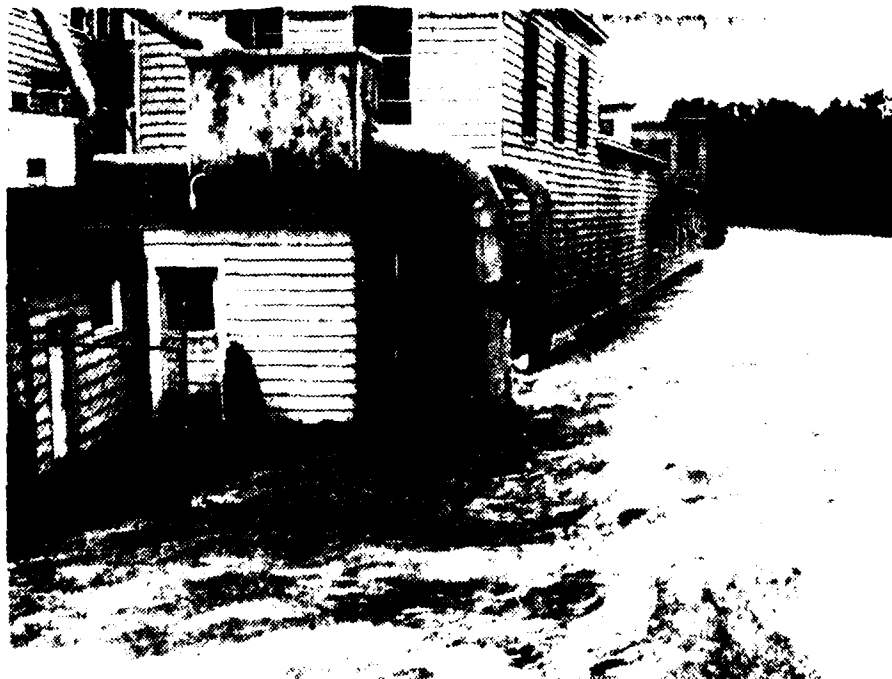
June 23, 1972 looking downstream at stream mile 7.1.
