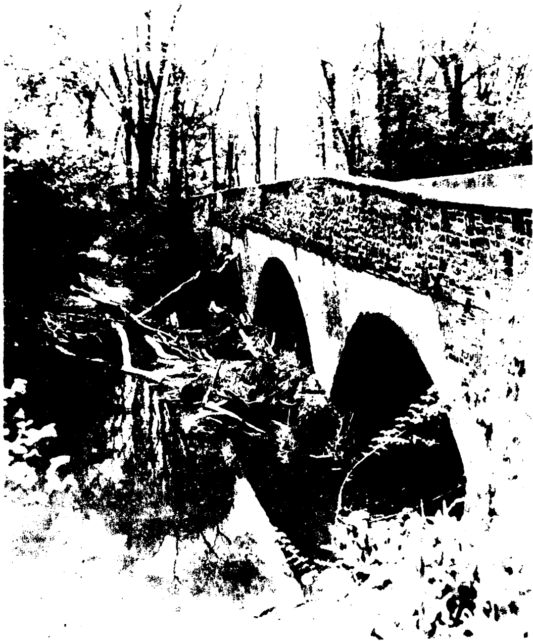
FIGURE 1 - Debris deposited at the Camp Road Bridge would be obstructive to floodflows.
