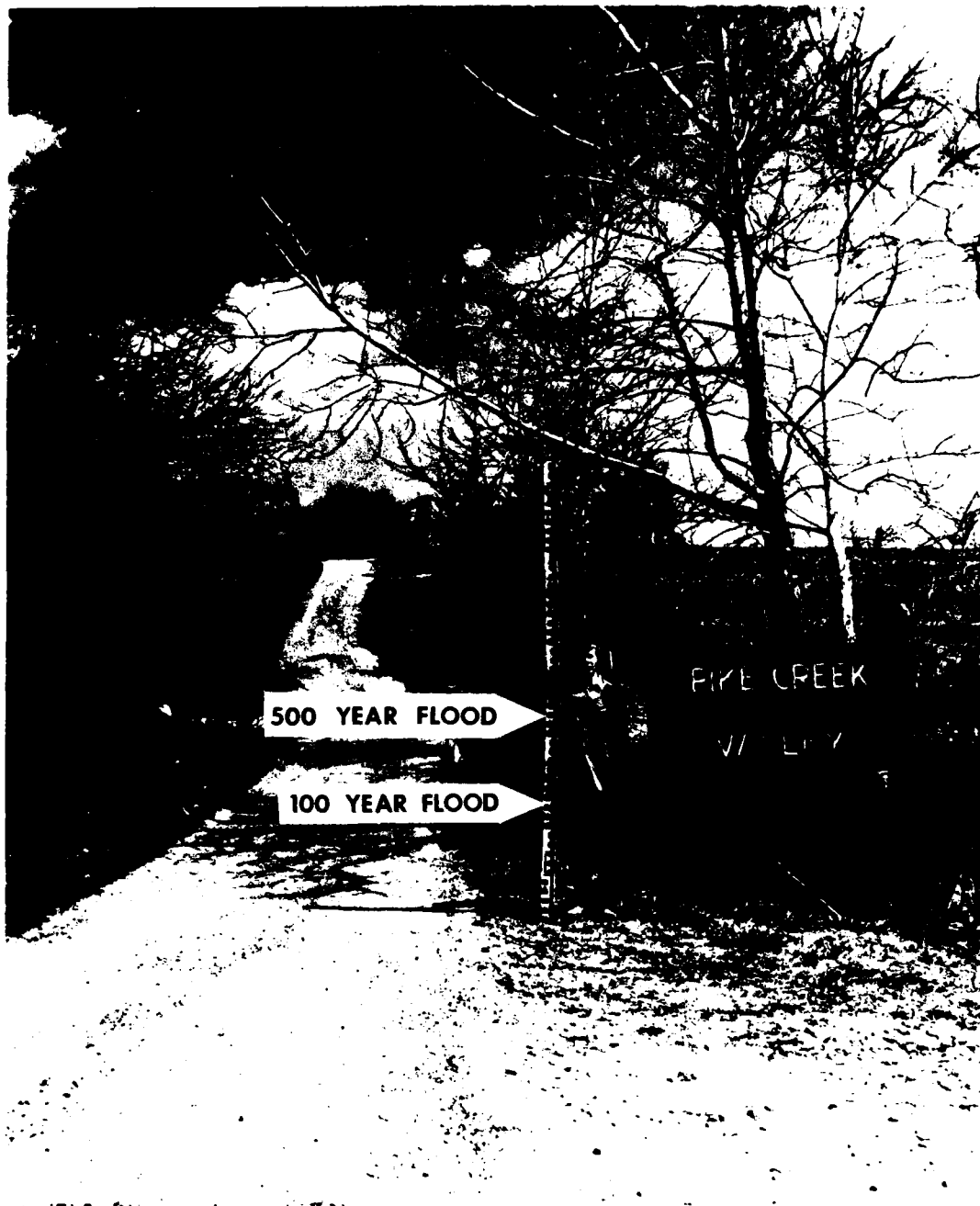
FIGURE 1 - Possible future flood heights at a Private Road Bridge (Mile 3.02) over Pike Creek.
