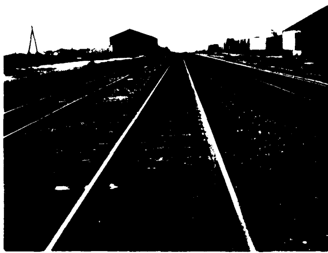
Figure 21. Castroville - Sidings - (Could be used for car storage or end loading of vehicles using portable ramps.)
