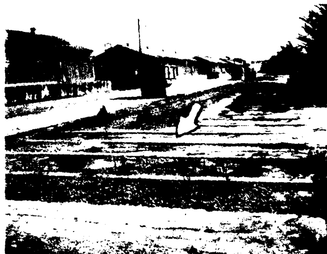
Figure 6. Spur 1033. (Note the existing concrete footings (arrow) for an end-loading ramp in the bottom photograph; top photograph shows hardstand and adjacent warehouses.)
