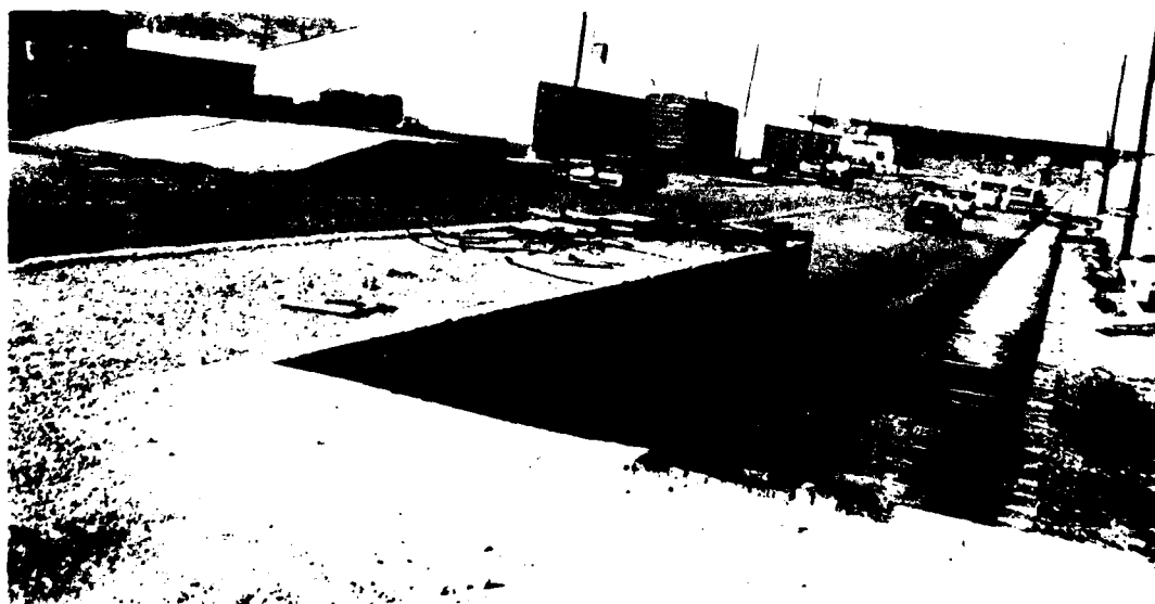
Figure 21. Concrete Ramps at Tracks 10 and 11 (Looking North).
