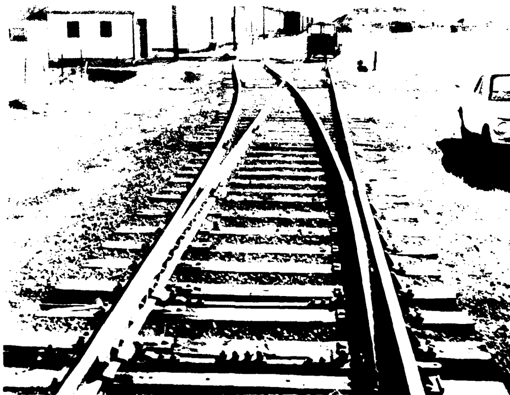
Figure 9. Tracks 4 and 5 (Looking South), Track 5 on Left.
