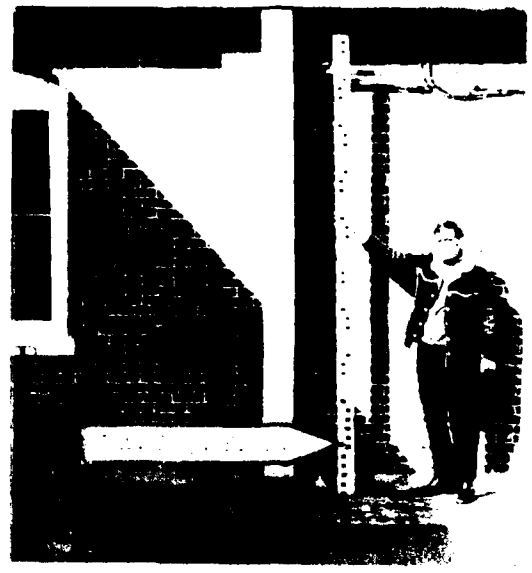
FIGURE 12 - Future flood heights at the Curtis Paper Co. on Chapel St. (Del. Rt. 72). The Standard Project Flood would be 3.3 feet above top of rod.
