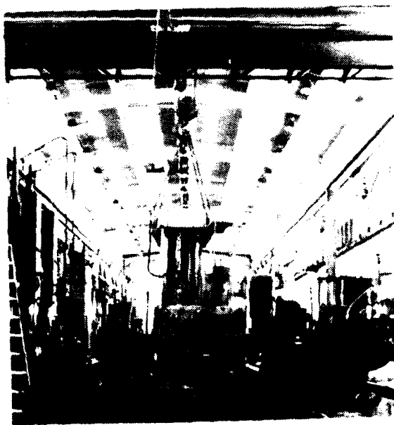
Bridge crane used for moving
