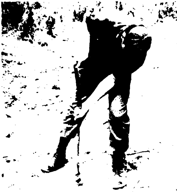
a. Hand augering using converted entrenching tool
