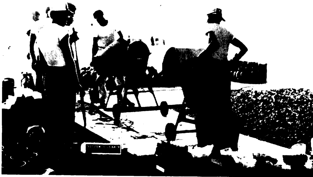
Figure 19. Mixing and Pouring Polymer Concrete, Test Item 35
