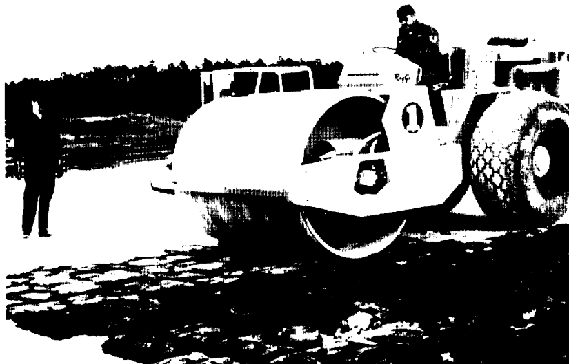
Figure 50. Compaction of Amalgapave®, Item 20
