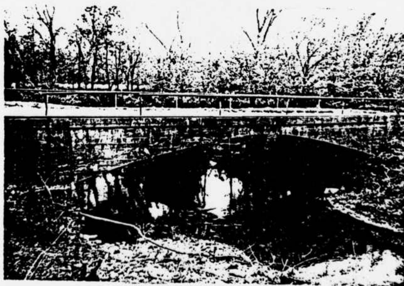
Figure 16. Bulls Creek and Snake Creek Bridges.
