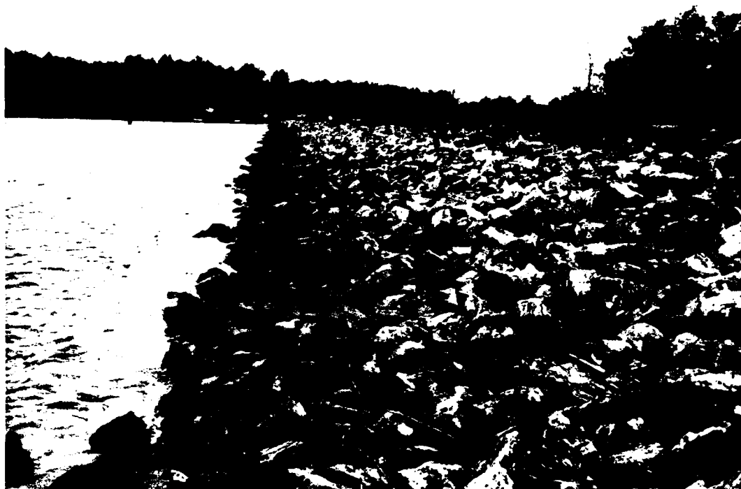
PHOTO 5. Riprap on Upstream Embankment, Emergency Drain Control and Support in Left Background
