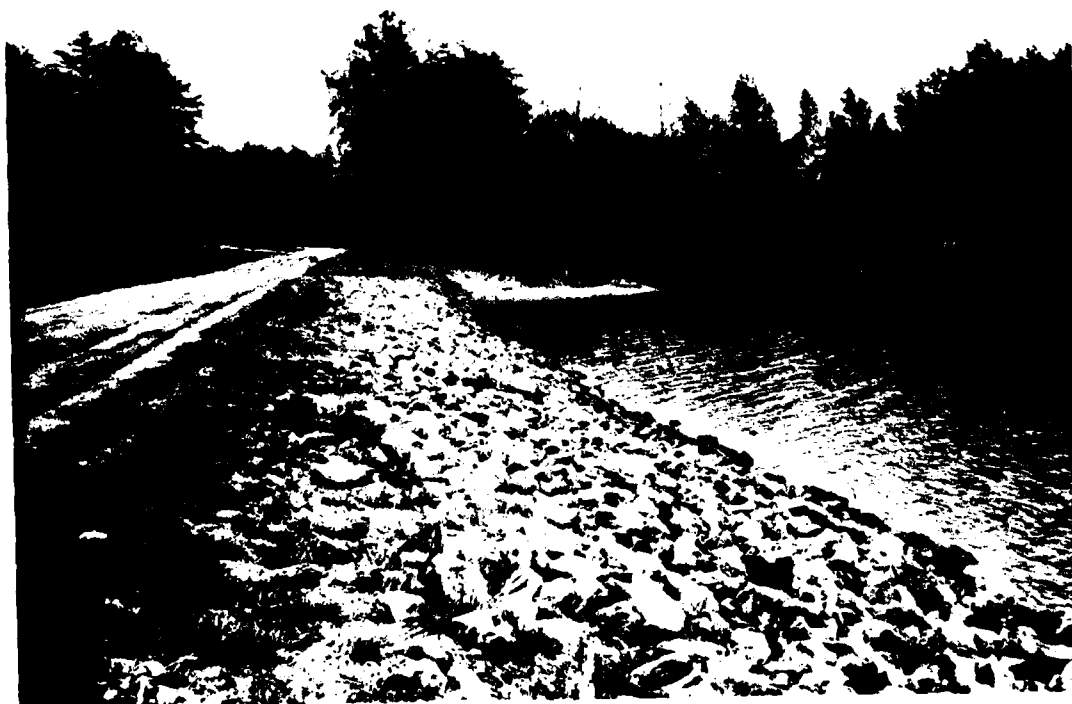
PHOTO 4. Right Abutment Area
