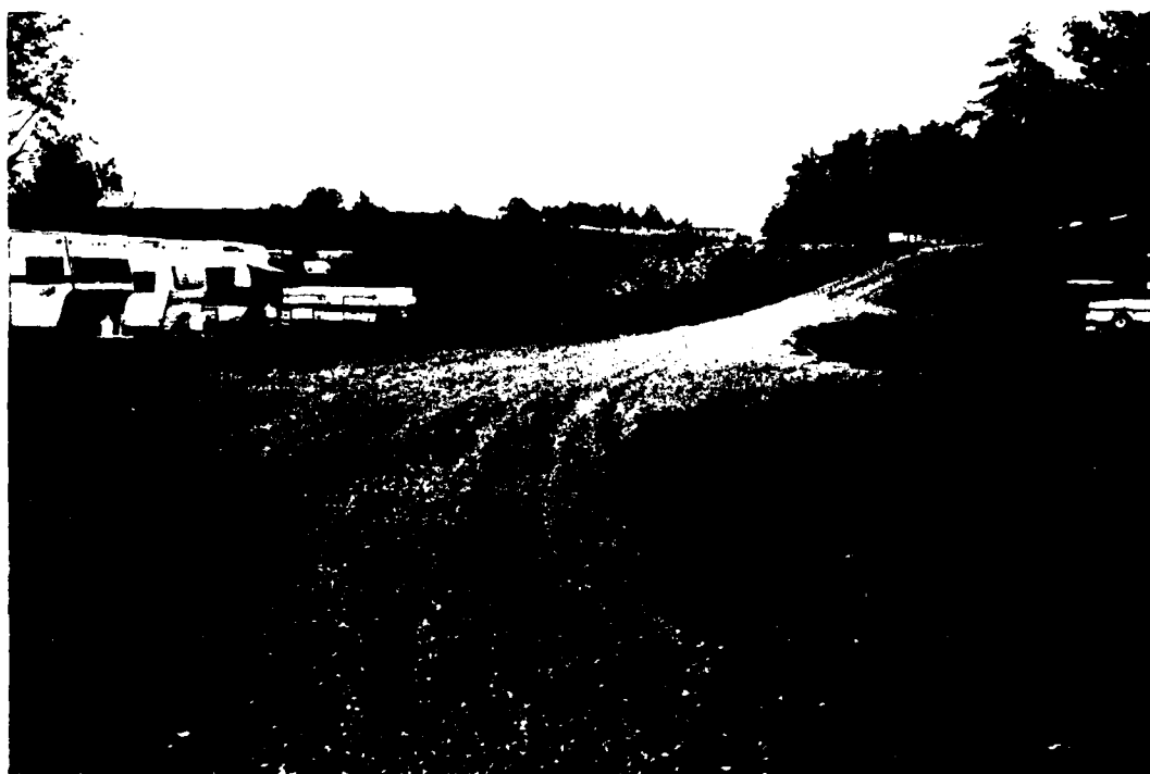
PHOTO 2. Camper Storage and Campground Immediately Downstream of Spillway
