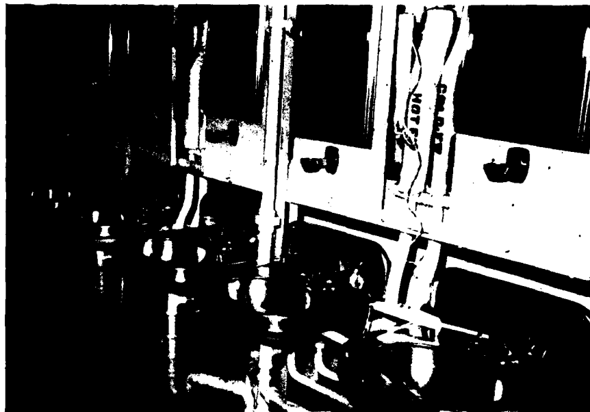
Figure 34. Typical Shipboard Lavatories, USS LEXINGTON (AVT-16)
