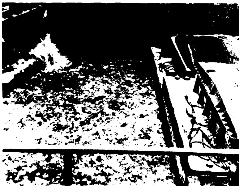
Figure 13. Lock clearance reduced by ice, Lock and Dam 26, Mississippi River.
