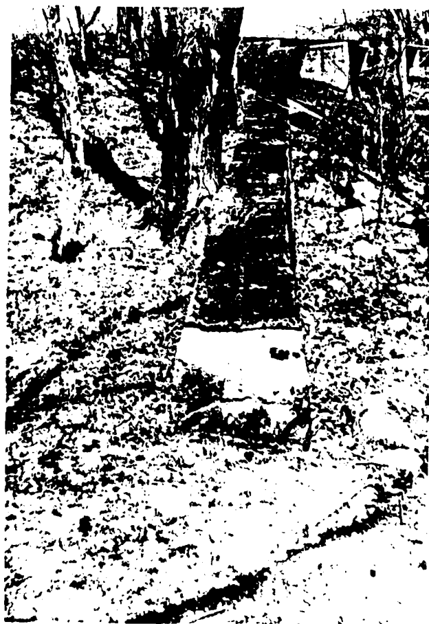
Right Spillway training wall running outward parallel to chute of spillway on downstream face of dam. Wall actually is for the spillway chute.
