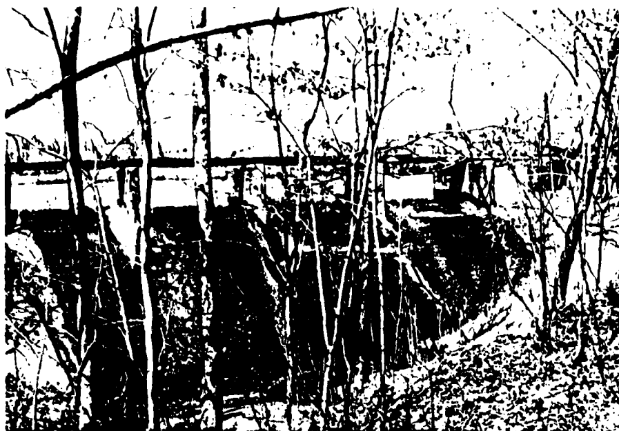
Downstream face of overflow spillway. Note repaired concrete at left (east) side (right edge of photo).
