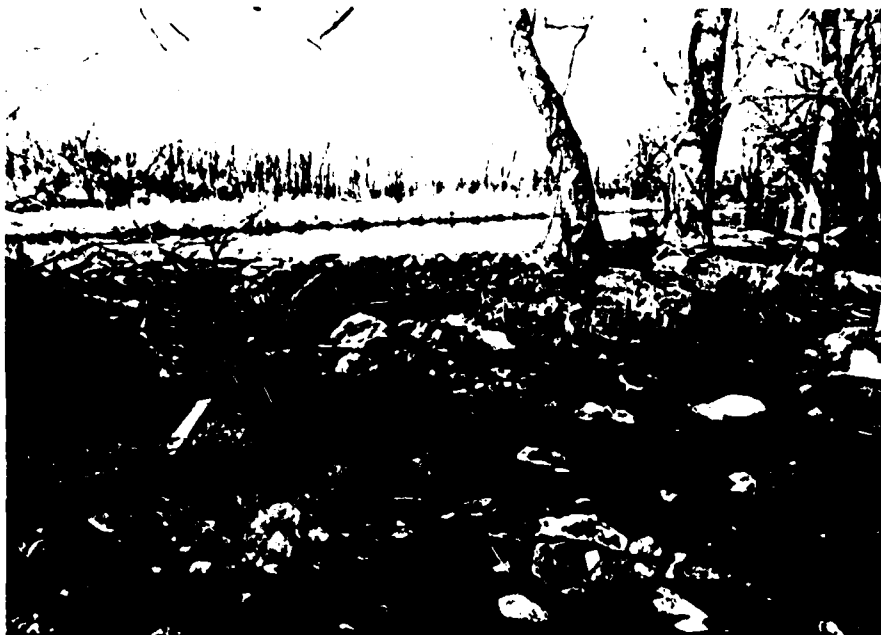
General appearance of dike - part masonry, concrete, concrete capping, and debris. Flow of water from under and through dike along most of its length.
