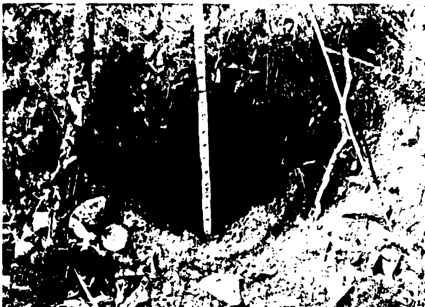
View of an animal burrow, 10 inches in diameter, 3.5 feet deep; located halfway down the dam embankment slope.
