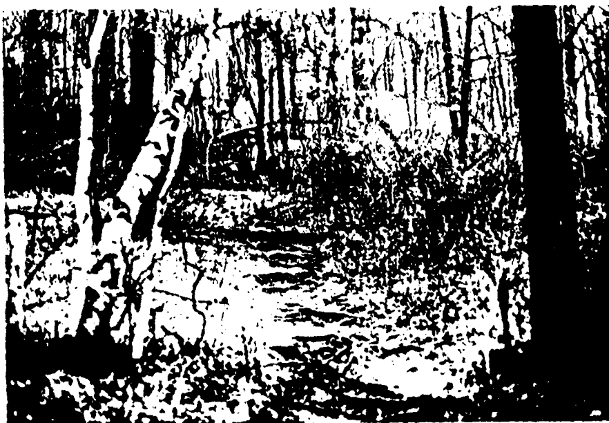
View of extensive root growth downstream of right side of dam.
