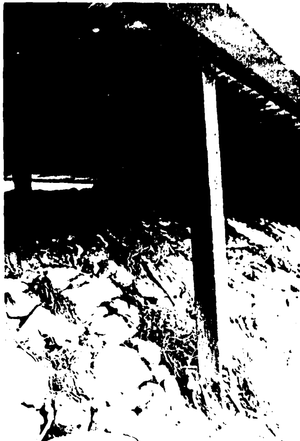
View of underside of road bridge over spillway; note that bridge column nearly rusted away at footing.
