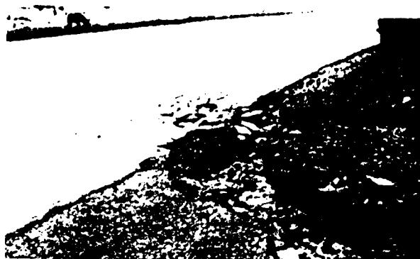
Erosion of shoulder by rain runoff from the road, with damage to pavement by headward erosion. Zone III/IV. Trucial Coast
