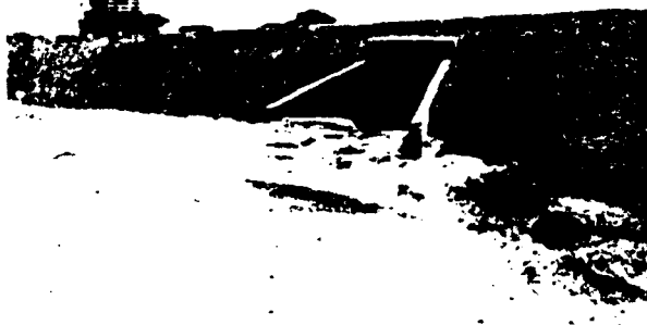
Erosion in granular fill behind unprotected culvert headwall due to streamflood conditions. Zone III Trucial Coast
