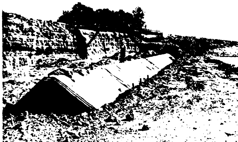
NO. 5: CURING SPILLWAY MONOLITHS
