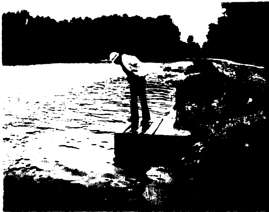
Photo 13: Culvert Control Structure at Section "E"
