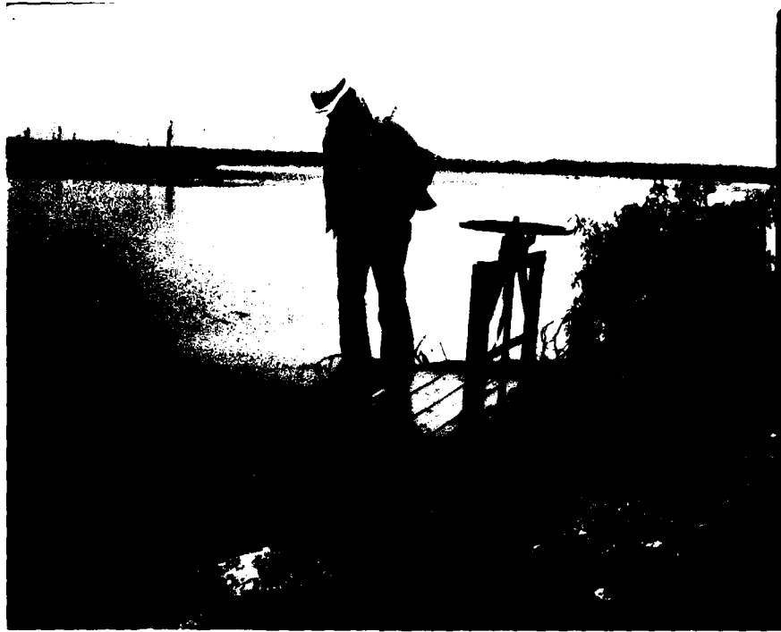
Photo 9: Culvert Control Structure at Section "Q"
