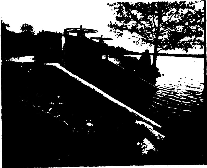
Photo 15: Sluice Gate at Section "H"
