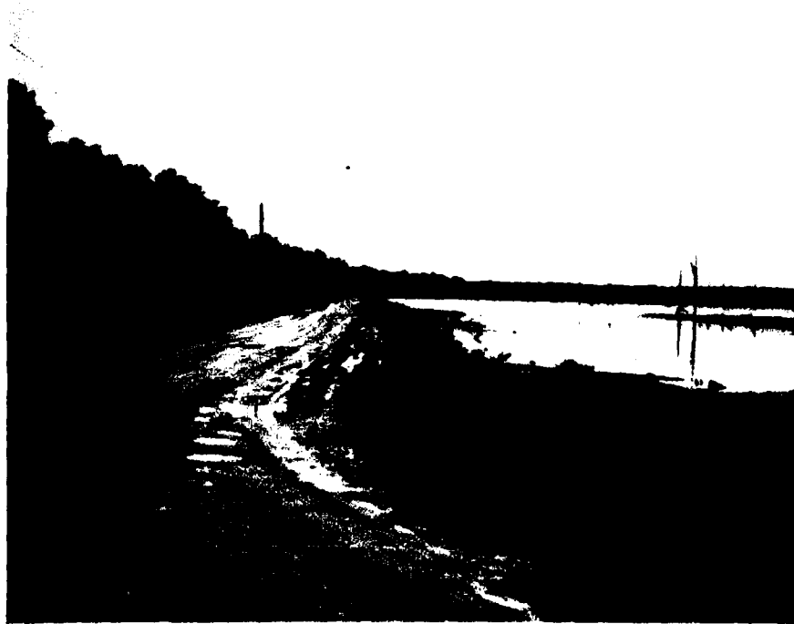
Photo 4: Southern Levee - Looking East to West
